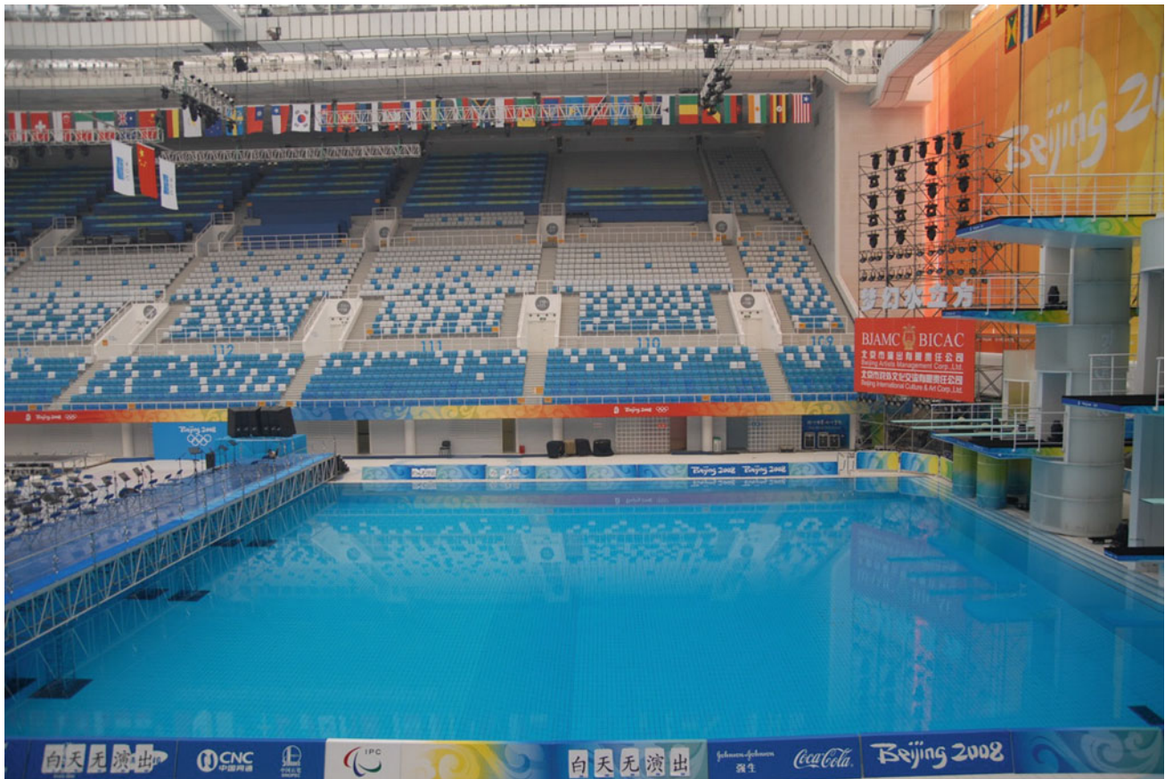
Fig. 10.66 “The Water Cube” (178 m 2 and 31 m high), National Swimming Center for Beijing 2008 summer Olympic Games, designed based on the spread pattern of cells and the natural structure of soap
