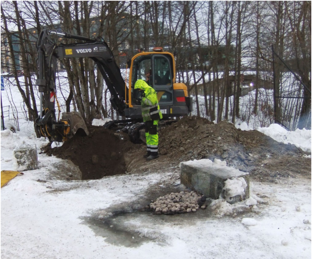
Fig. 3.16 Digging ditches in the winter. The machine must cut through the hard frozen top layer. Here they have made a small fire with coal to melt the frost and ease the digging operation
