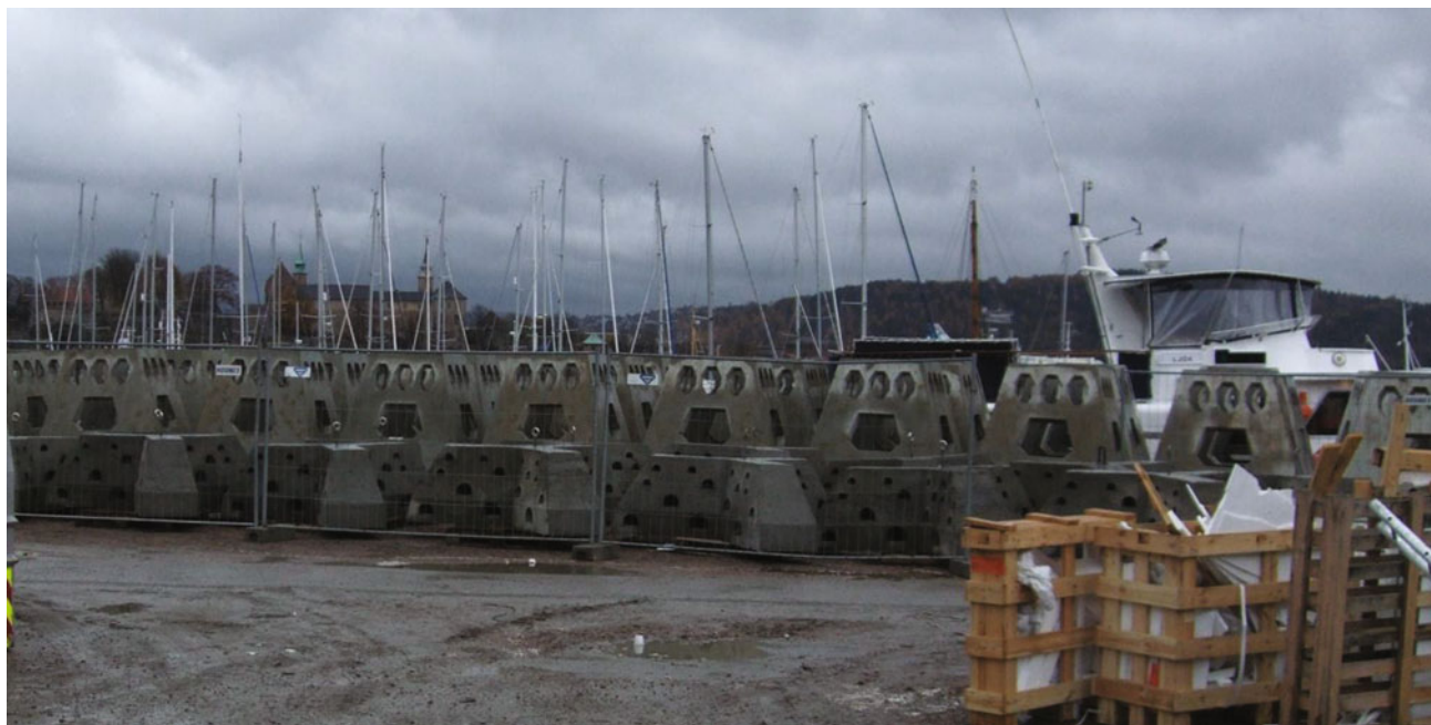
Fig. 11.59 Reef modules in the harbor, ready for placing in the sea
