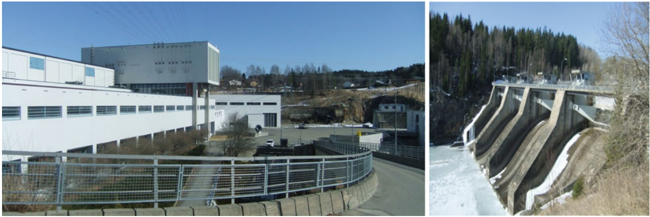
Fig. 7.16 Kykkelsrud power station in Glomma (Norway's longest river) in Askim community in Østfold County utilizes a fall of 26.5 m and is owned by the company Hafslund. The power station is rehabilitated and was reopened in April 2011 with a capacity of 40 MW [18]. The power station was originally started 1900 and taken over by the company Hafslund in 1915. Before the reconstruction the station
