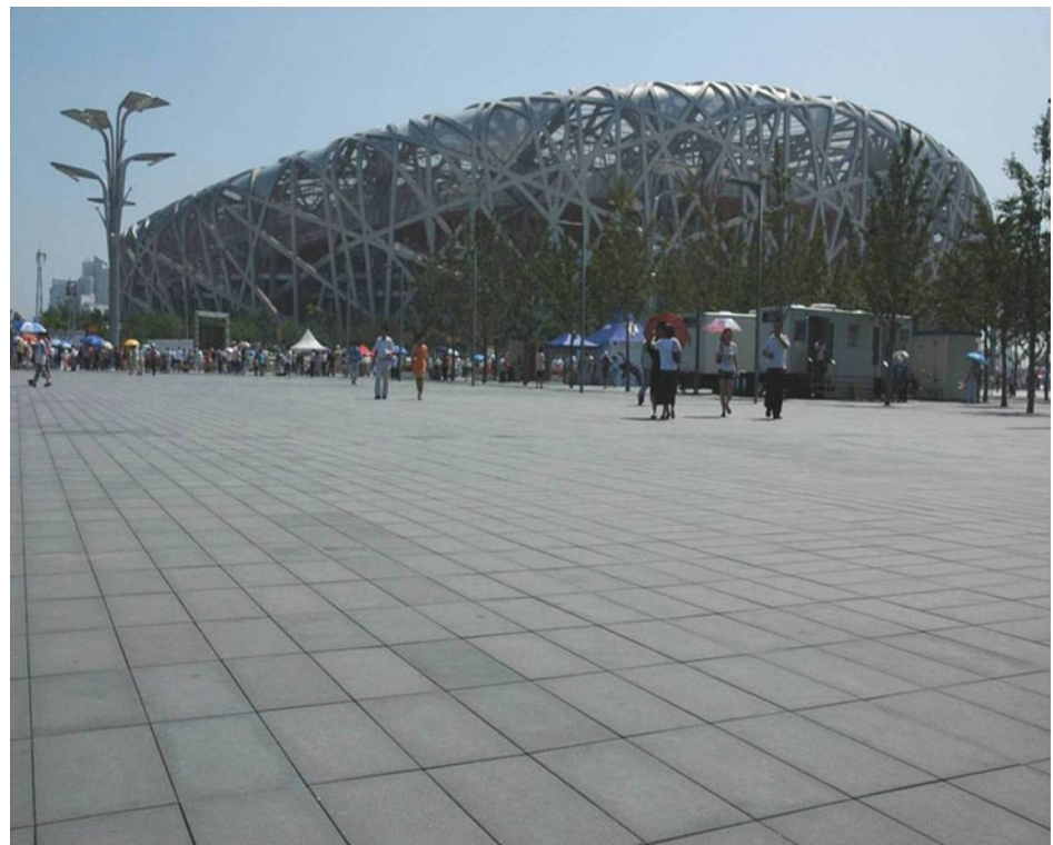
Fig. 8.4 Permeable ground slab outside the Olympic stadium “the Birds Nest”, Beijing, China
