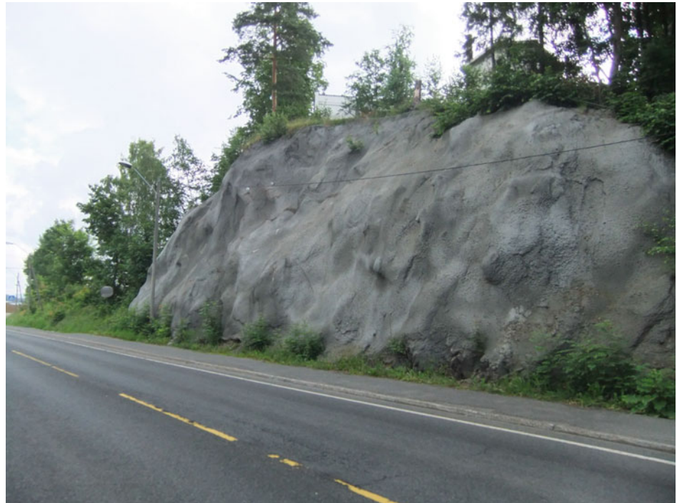
Fig. 8.25 Rock cut protected by sprayed concrete, Old Drammen Road, Sandvika, Norway
