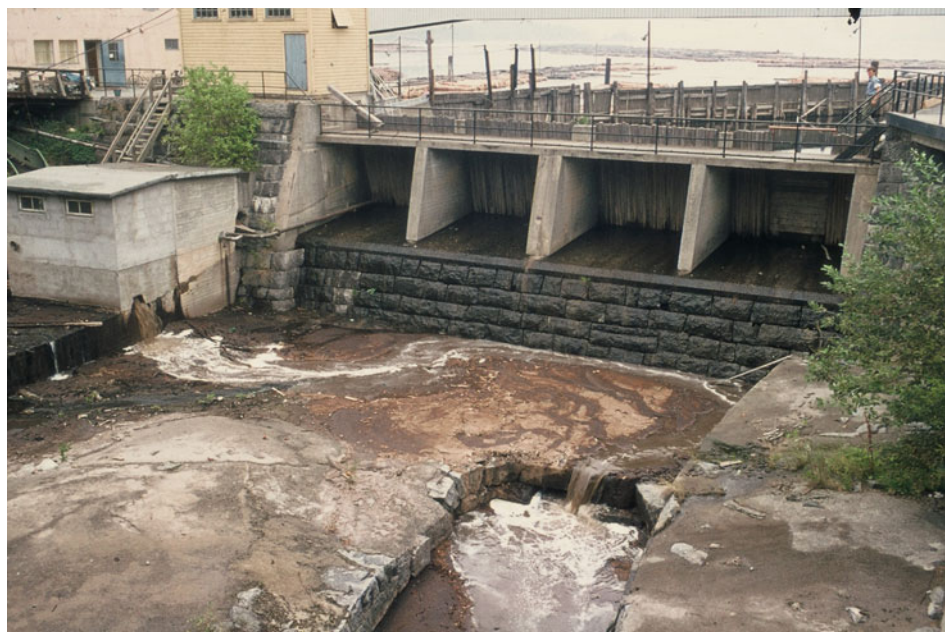
Fig. 7.18 The first time concrete was used in Norway was in the Farris Dam in 1764. The main purpose of the dam was to secure the town from more flood accidents
