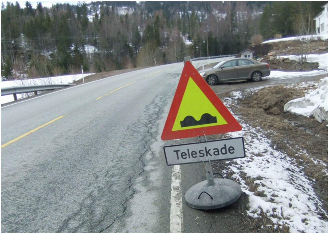
Fig. 8.27 Not an unusual spring message from the Road Department (Teleskade = Frozen ground damage)
