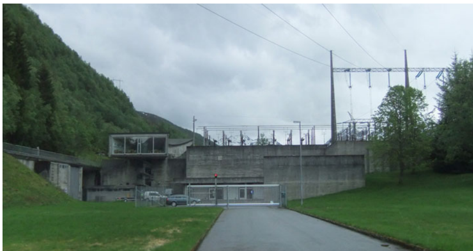
Fig. 7.15 Røldal Power Station, designed by Arkitekt Geir Grung in 1964. Geir Grung have also designed the station at Nesflaten, in the same power complex. That building is ranged as number 7 among Norway's most important buildings The waterfall power development
