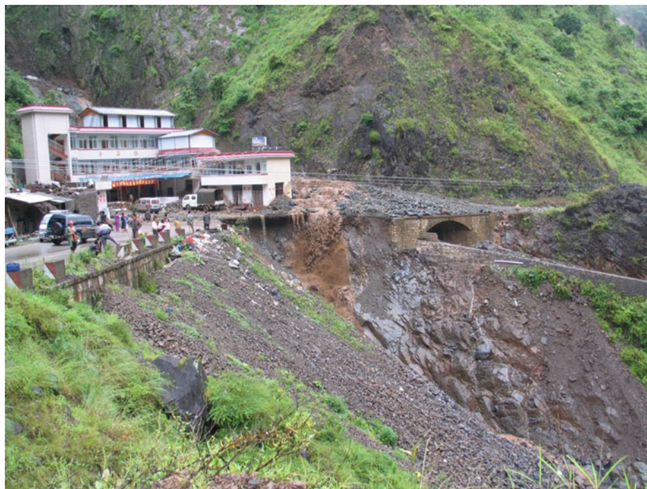
Fig. 8.6 Road between Yongsheng and Lijiang, Yunnan Province, China destroyed by landslide after heavy rain, September, 2004
