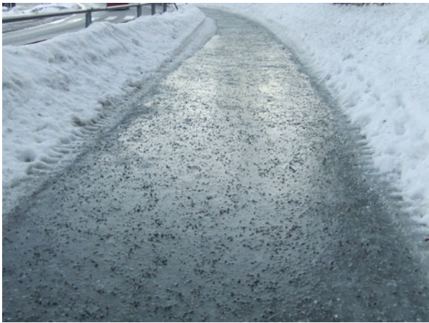
Fig. 3.6 Snowfall, rain and frost in a few days give a dangerous surface on the walkways
