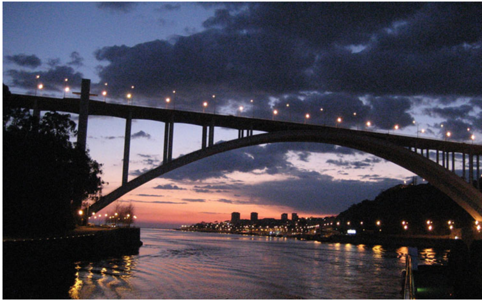
Fig. 5.38 A high bridge is crossing the Duero River in Portugal between the cities of Porto and Gaia. The many rivers in the world are a true gift and a great challenge to bridge engineers. Many of the bridges that have been designed and constructed have got great attention because of their elegance and engineering wise adjustment to acceptable esthetic norms
