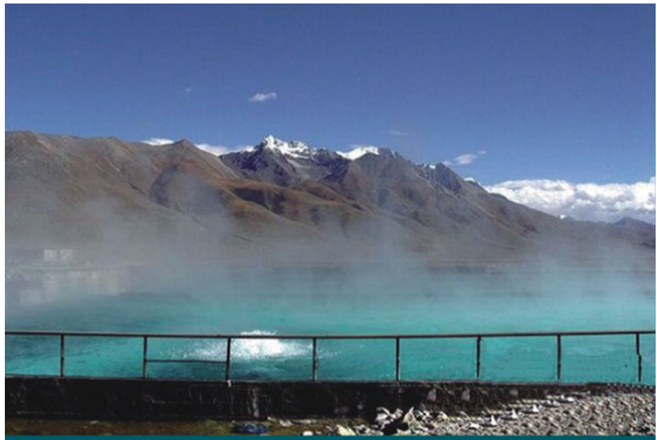
Fig. 7.14 Yangbajing geothermal field for power generation, located in Dangxiong County, 91.8 km Northwestern Lhasa, Tibet, Western China
