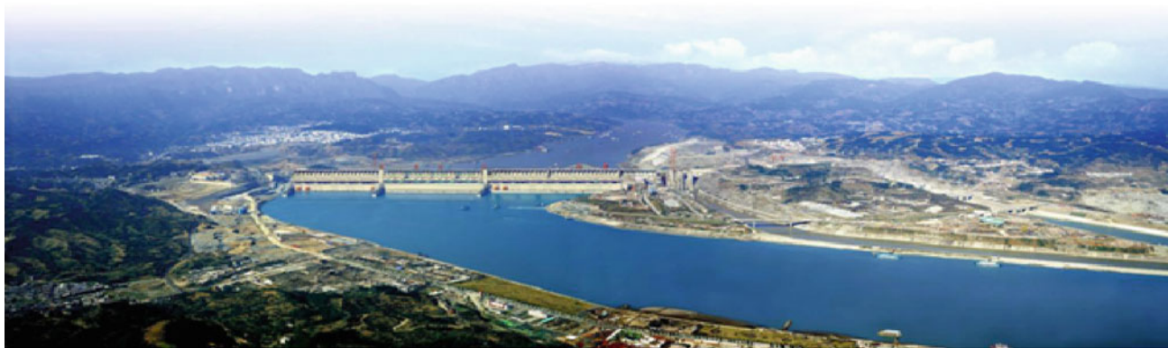
Fig. 7.20 The Three Gorges Dam was built from 1993 to 2009. The power station equipped with a total installed capacity of 32 \times 700 MW produces every year 100 billion kWh. The huge concrete gravity dam
