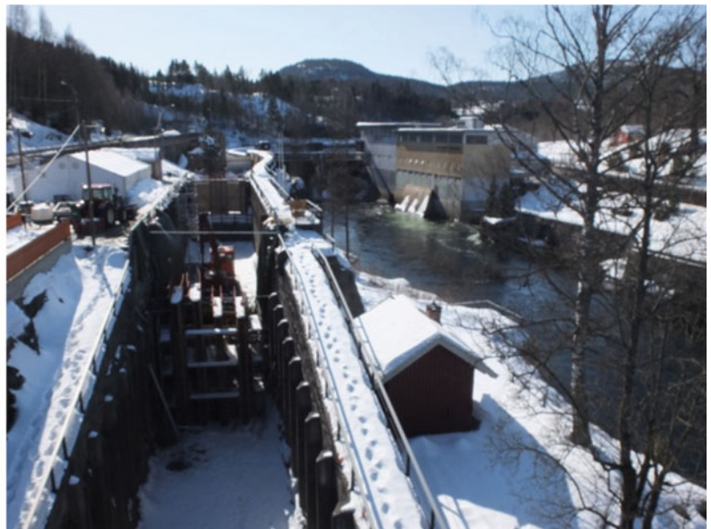
Fig. 6.13 Vrangfoss locks and Ulefoss locks. Repair and maintenance of the locks must take place in the winter months
