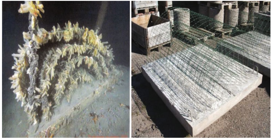
Fig. 11.57 Cleaning reef modules after half a year on the bottom ( left ) and before setting out ( right )
