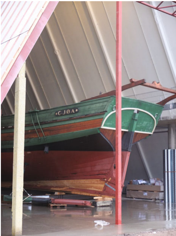
Fig. 3.4 Autumn 2012—A house is built around “Gjøa” at Bygdøy in Oslo
