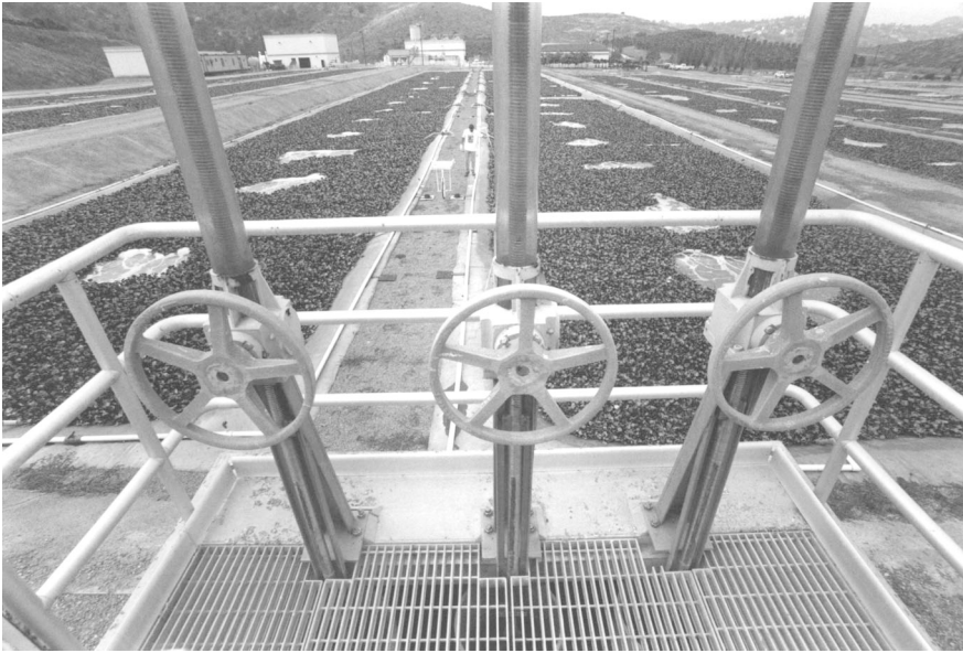
Channels containing water hyacinths, used to provide secondary treatment at San Diego's Aqua II pilot facility. Photo by Joe Klein.
