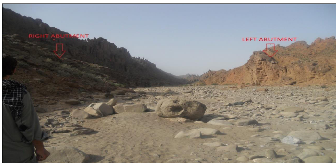
Figure 17 - Right & Left Abutments of Siri Toi dam
