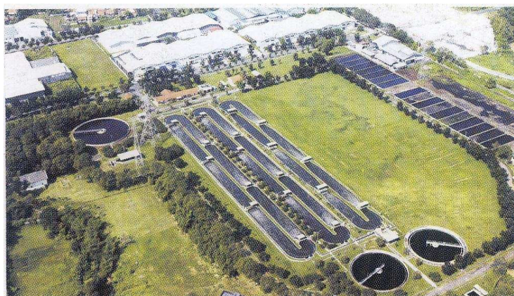
Figure 1. Jababeka Wastewater Treatment Plant
