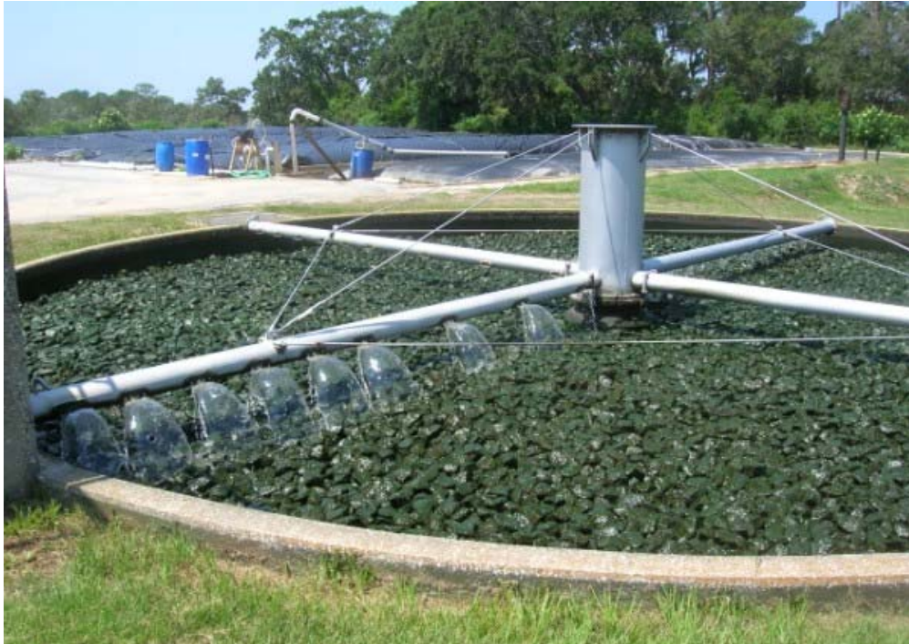
Figure 1 Circular trickling filter gravel pack (from http://www.purewatergazette.net ).
