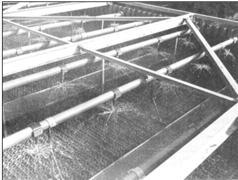
Figure 3.- Left: Fixed wastewater distribution system. Right: Mobile wastewater distribution system of rotating arms on circular beds ( http://www.enviopro.co.uk )
