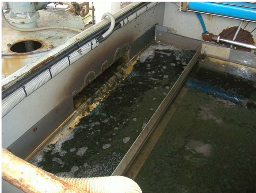
Figure 16. General view of the feeding área of a band filter.
