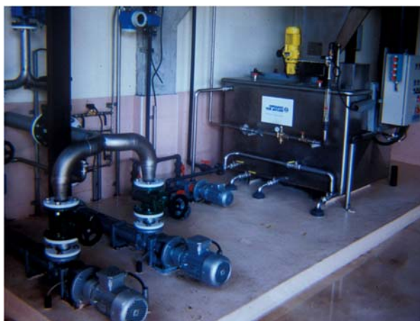
Figure 2 Compact equipment for polyelectrolite preparation in sludge conditioning.
