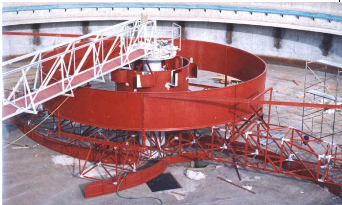
Figure 20 Double-baffle central feeding system
