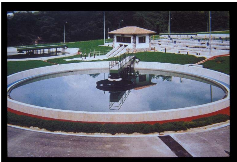
Figure 12 General view of a circular primary clarifier with moving arm.
