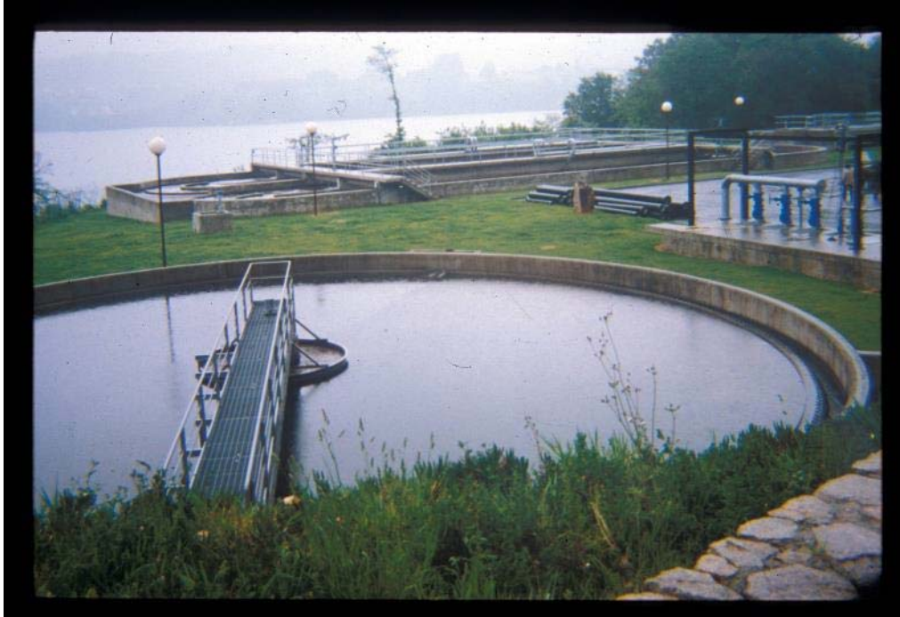
Figure 13 General view of a circular primary clarifier with moving arm.
