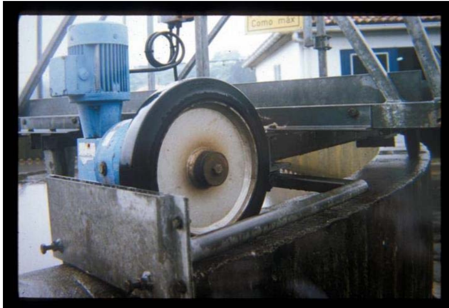
Figure 17 Drive unit of a circular clarifier moving arm.
