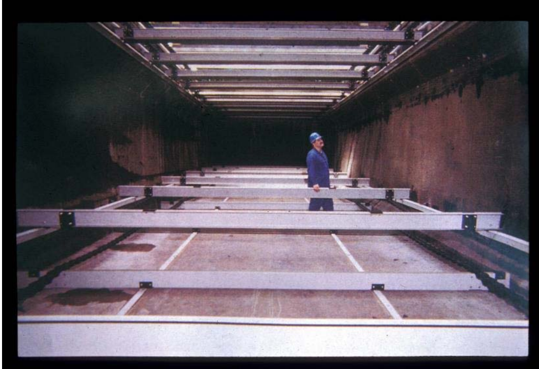
Figure 5 Detail of sludge and scum extraction system by chain scrapers and skimmers
