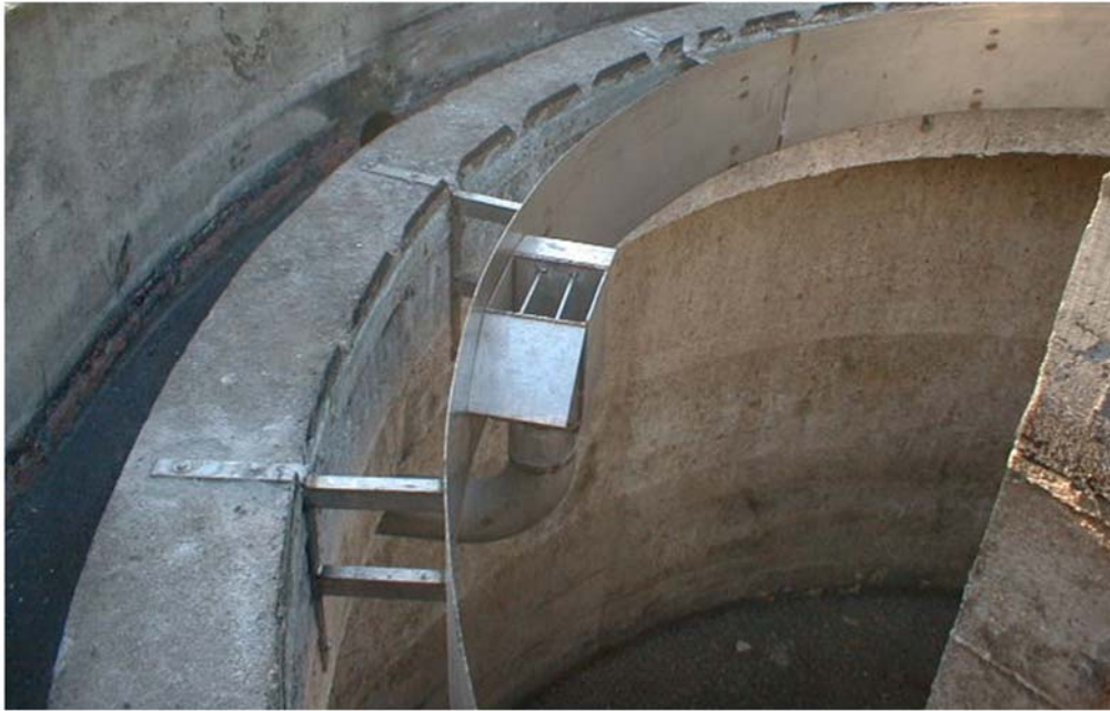
Figure 7 Detail of a scum trough on a primary clarifier
