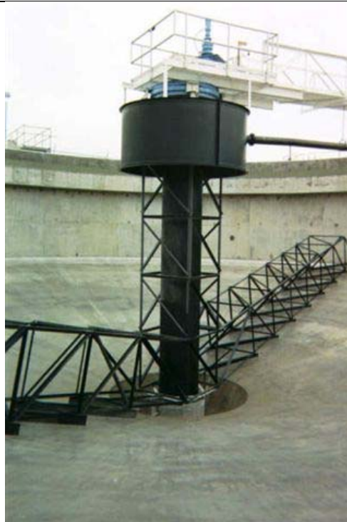
Figure 30 Bottom scrapers system fixed to central drive unit.
