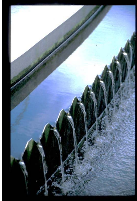
Figure 23 Detail of clarified water over the effluent weir: baffle and v-notch weir.
