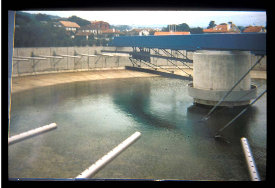
Figure 25 Clarified water extraction system by radial perforated tubes
