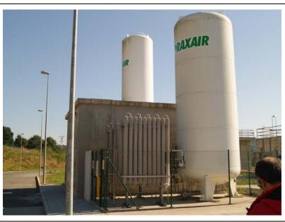
Figure 1.- Cooling system and oxygen storage (ETAP-Lugo).
