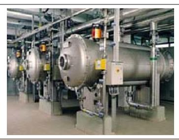
Figure 6.- Horizontal ozone generators at industrial scale.
