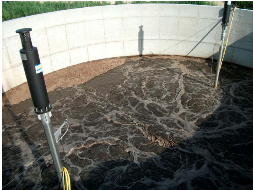
Figure 10 General image of a regulation-homogenization tank.
