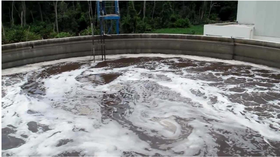
Figure 9. General image of a regulation-homogenization tank.
