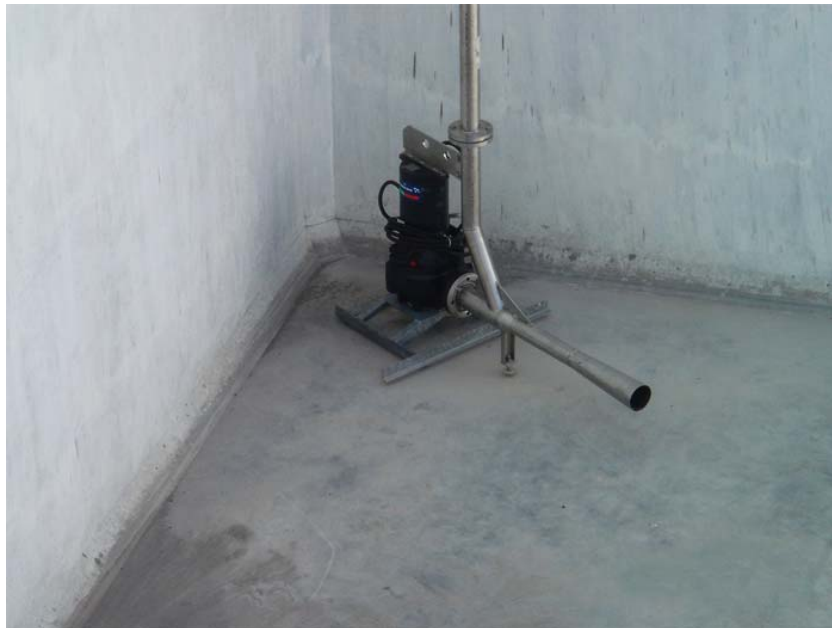
Figure 4 Agitation system ejector example
