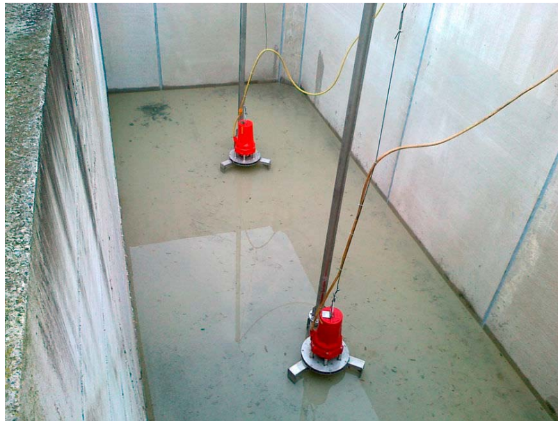
Figure 5 Bottom agitation system
