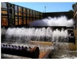
Figure 5-3: Example of spray aeration at Western Australian Groundwater Treatment Plant
