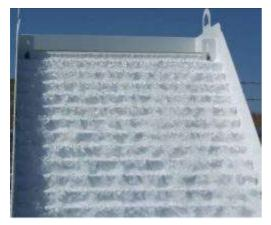
Figure 5-4: Example of cascade aeration unit
