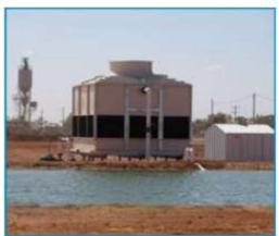
Figure 5-5: Proprietary Lakeside cooling tower treating (cooling and aerating) bore water
