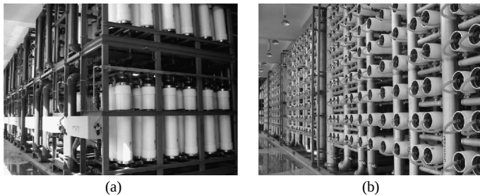
Figure 4.6 Full-scale integrated membrane system (IMS) of Caotan water purification plant for tap water supply located at Kaohsiung County, Taiwan (a) Ultrafiltration system; (b) NF-LPRO system. The total land area of IMS is 1380 \text{m}^2 . (Photos provided by KINTECH Technology Co., Ltd.)
