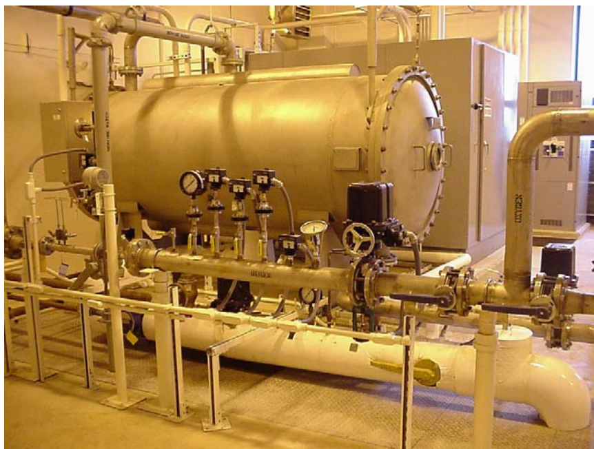
Large Ozone O_3 generator. We will see more and more of tri-oxygen generation.
