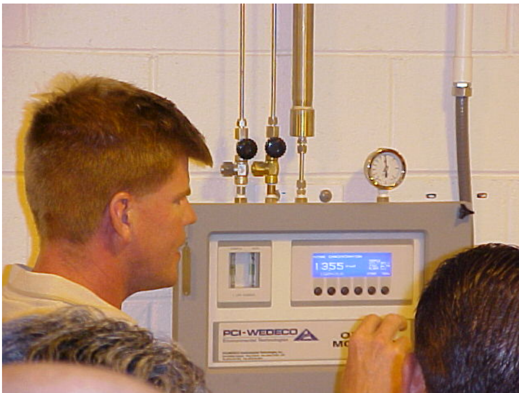
Ozone generator and control panel.
