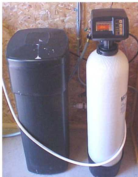
Softener with brine tank on right
