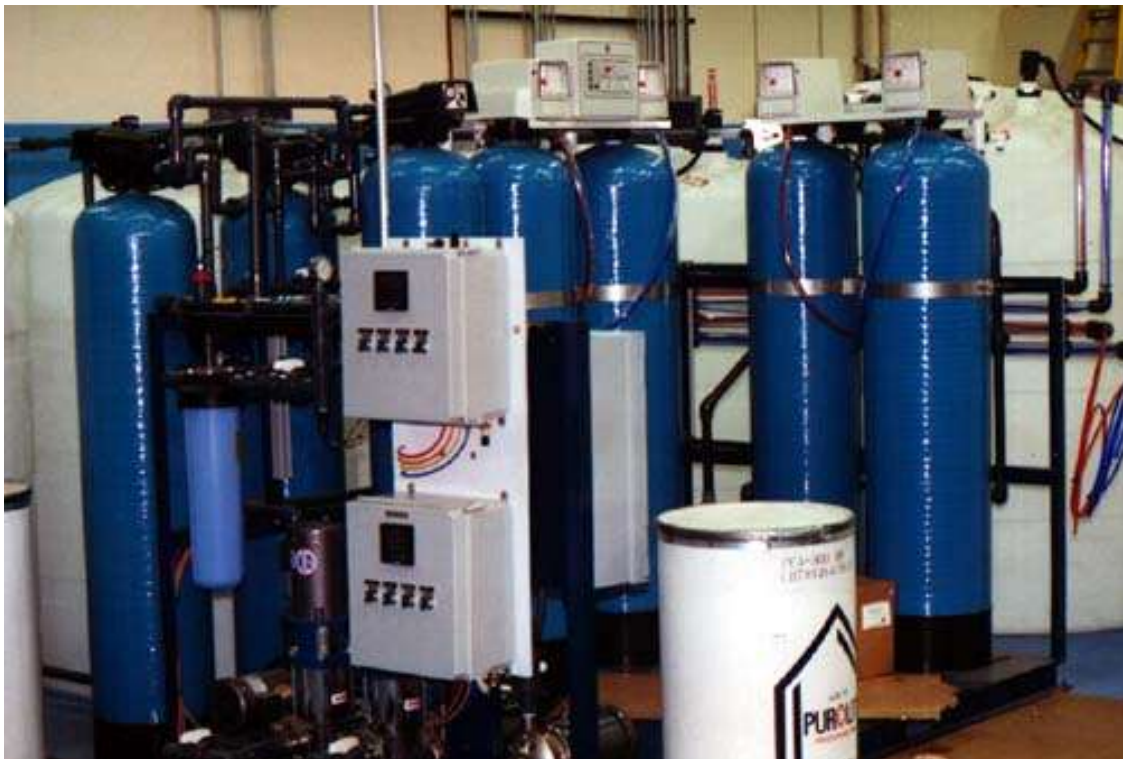
Ion Exchange Units
