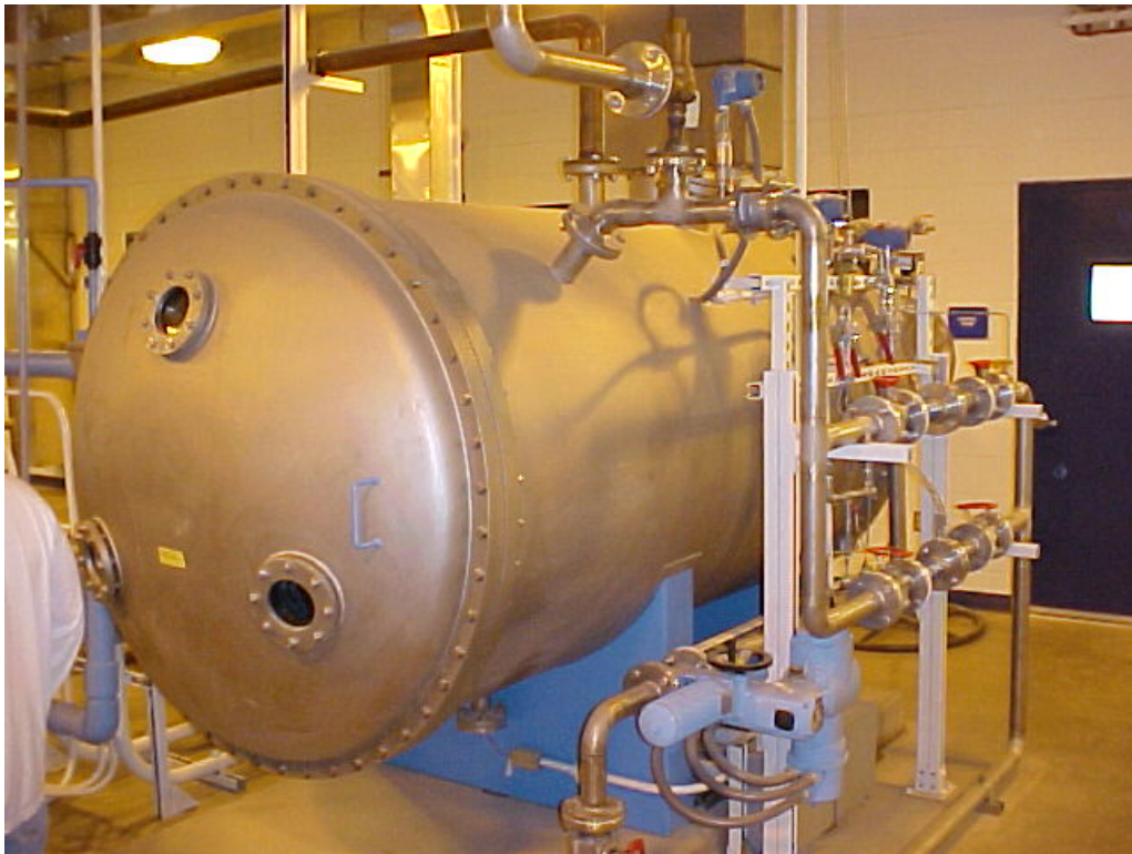
Ozone generator and control panel.
