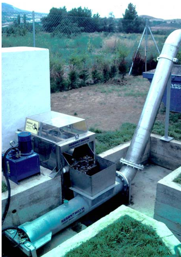
Figure 29 Piston based waste drive system and compaction
