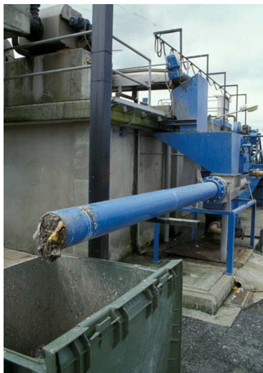
Figure 28 Waste drive system and compaction based on Archimedes screw
