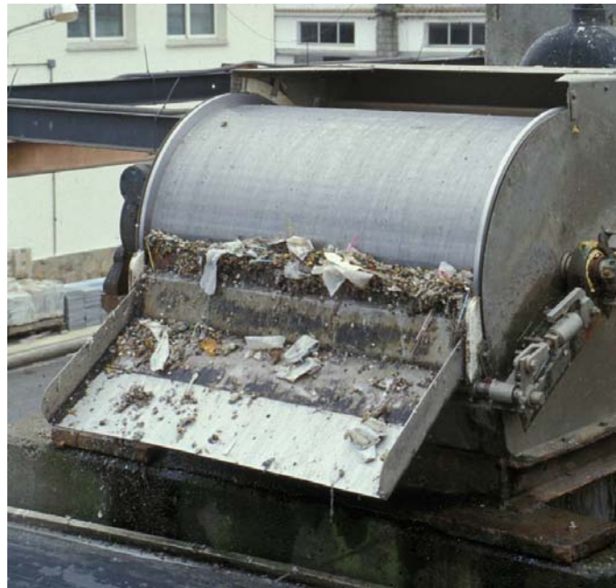
Figure 19 Rotary screen waste outlet detail
