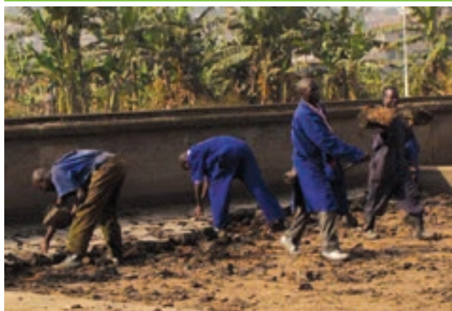
FIGURE 5. MANUAL SLUDGE REMOVAL FROM A DRYING BED (SLUDGE DRYING BEDS AT A SEWAGE TREATMENT PLANT, BUGOLOBI, KAMPALA, UGANDA).
