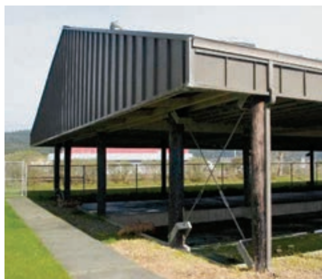
FIGURE 3. TYPICAL COVERED DRYING BED.
