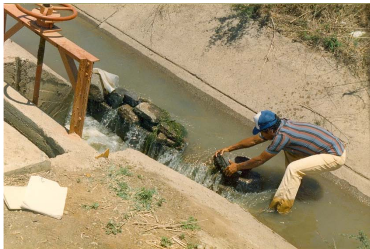
A water bailiff in a Mexican irrigation scheme changes the course of the water flow
