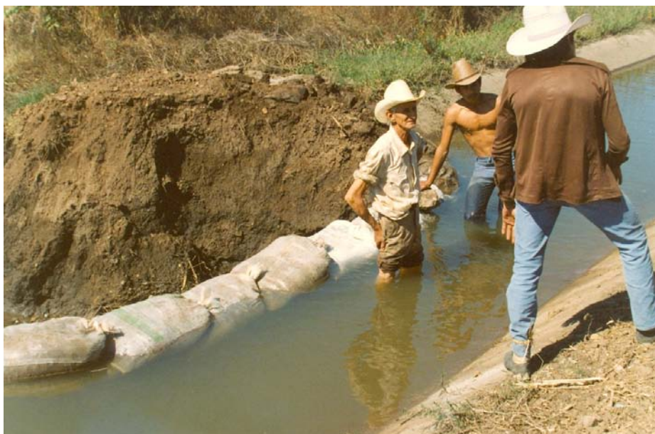
Irrigators repairing a canal in Mexico
