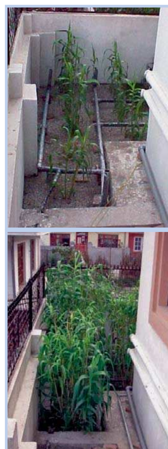
Photo 5-6: Vertical-flow planted filter shortly after completion (above) and in use (below) (photos: Shrestha R.R.)
