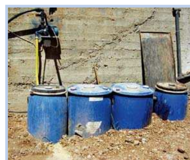
Photo 4-5: Four-barrel up-flow anaerobic filter implemented in Jordan. Two tanks of 220-litre capacity each filled with gravel media acting as anaerobic filters are inserted between a sedimentation and a final storage tank (photo: Redwood M., IDRC)
