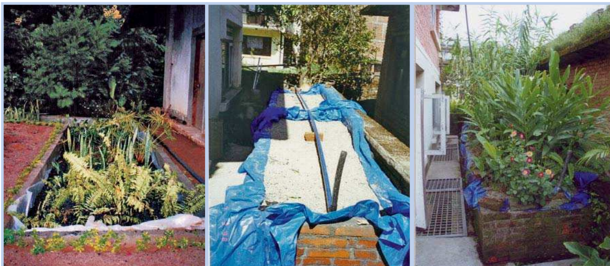
Photo 4-9: Left: VFPF treating kitchen and laundry greywater in a hotel in Sri Lanka, after pretreatment in a grease trap and septic tank (photo: Harindra Corea E.J.)
