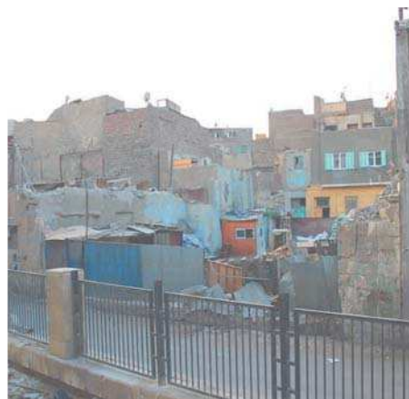
Fig. 4 Degraded buildings in El-Gamaleya
