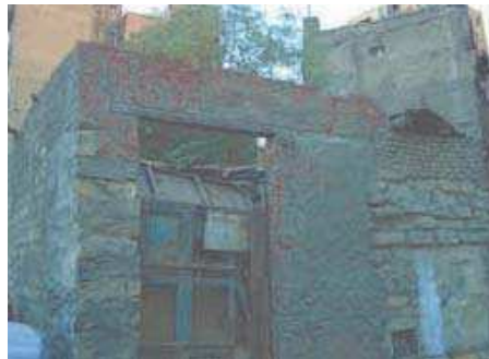
Fig. 3: Load bearing walls
