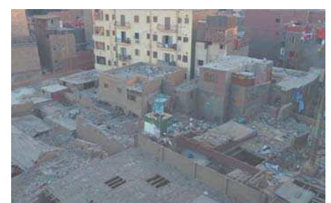
Fig. 3: Roof tops in El Gamaleya
