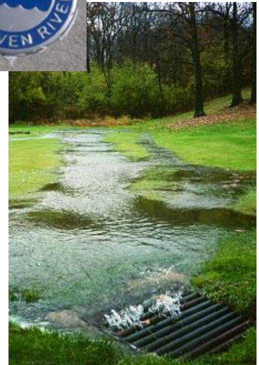
Runoff flowing into a stormwater drain.
