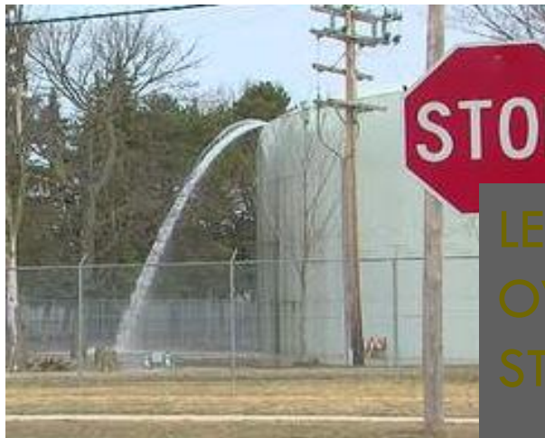
LEAKAGE ON MAINS
