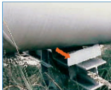
Fig. 1-b: Destroyed support (double T profile 200 mm, permanently deformed)
