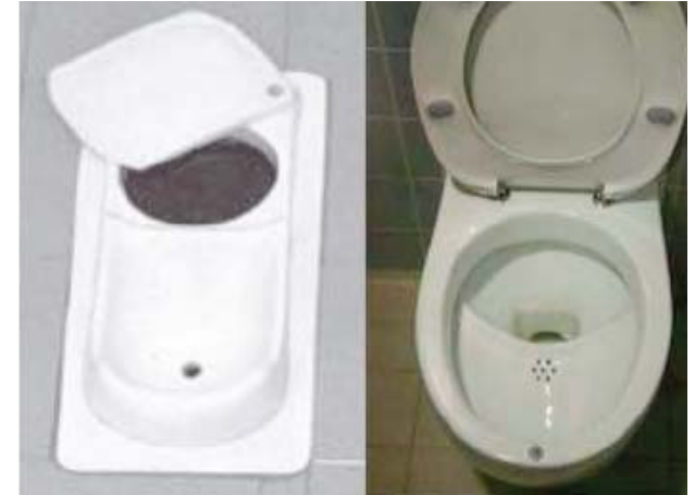
Urine separation devices [Right photo from WHO with permission (2006); left from Kvarnstrom et al., 2006]
