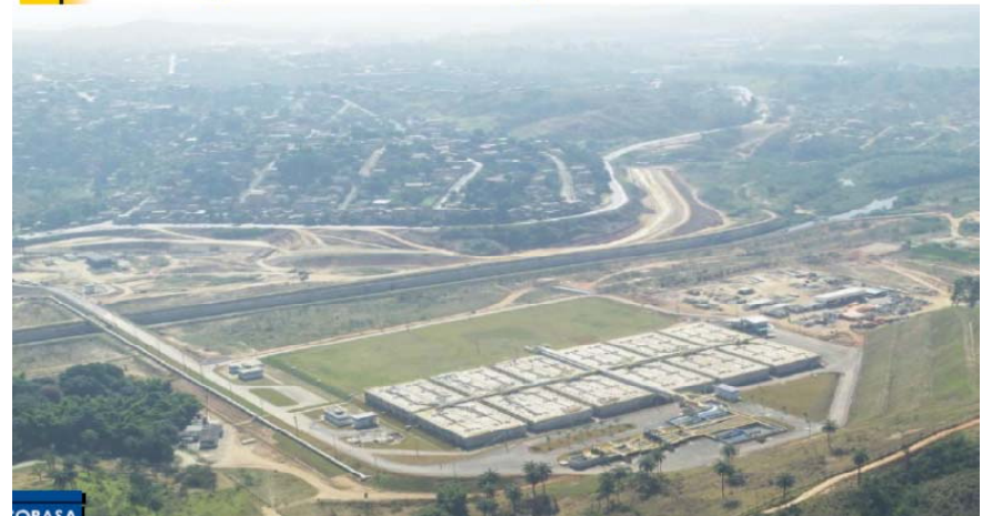
The Onca UASB Treatment Plant, Belo Horizonte, Brazil, Designed to Serve a Population of 1 million
