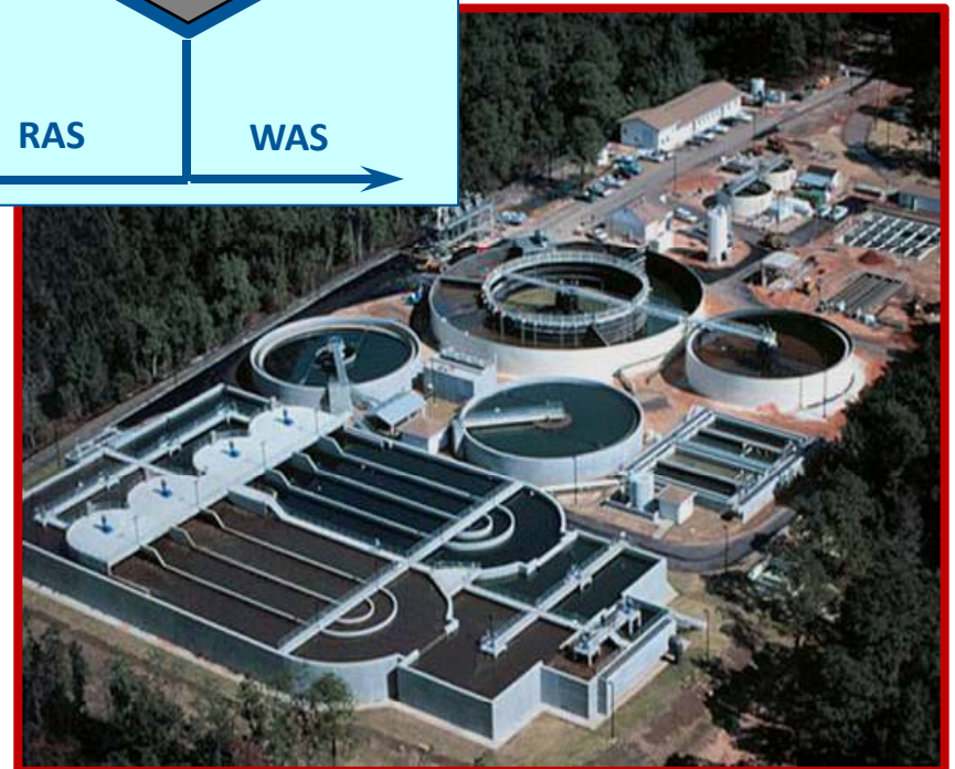
Bayou Marcus WRF Pensacola, FL
