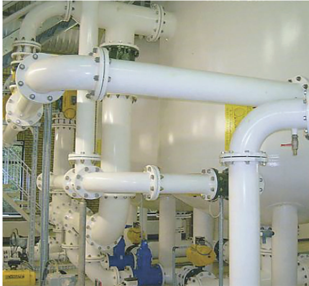
Figure 13 Rapid sand filters in groundwater treatment (Buamah, 2009)
