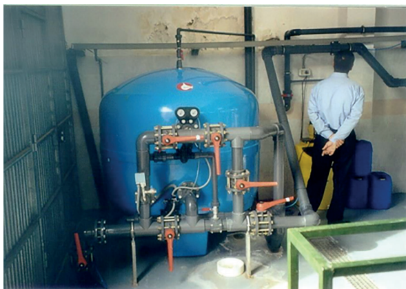
Figure 17 Sand filter. Gran Canaria, Spain.
