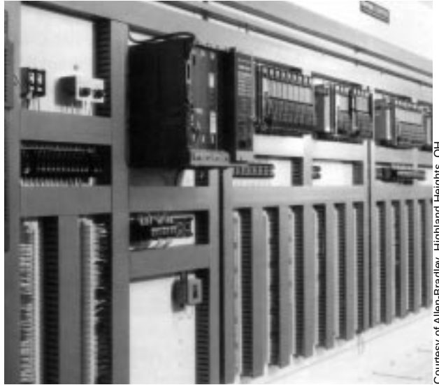
Figure 3. Placement of PLC components.
