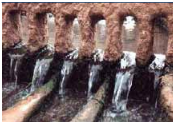
Figure 6.3 Water-Dividing Structure in a Foggara, Algeria
