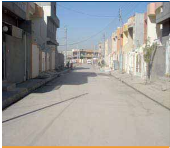
Figure 10.4 Badawa after Completion of Rehabilitation Works
