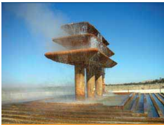
Figure 9.1 Cooling Tower Bringing Geothermal Water from the Sahara Down to a Temperature Usable in Irrigation
