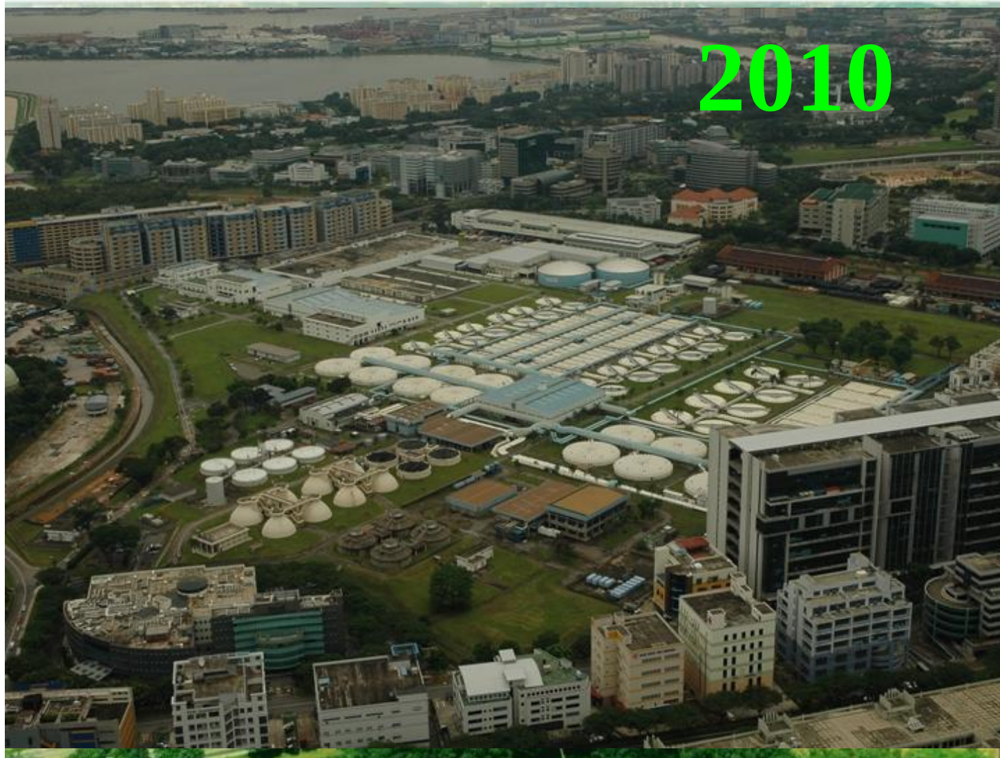
Ulu Pandan Water Reclamation Plant
