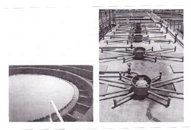
Figure 3.- Influent distribution structures in: (a) a circular reactor (left side) and (b) a rectangular reactor (right side).
