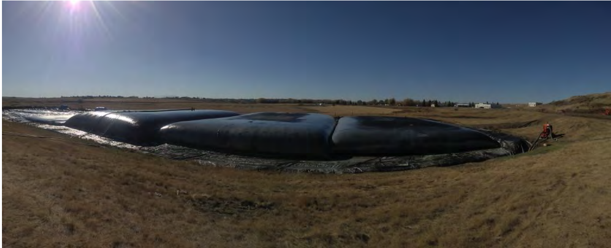
Figure 3-3 Lagoon De-sludging Using Geotextile Containers
