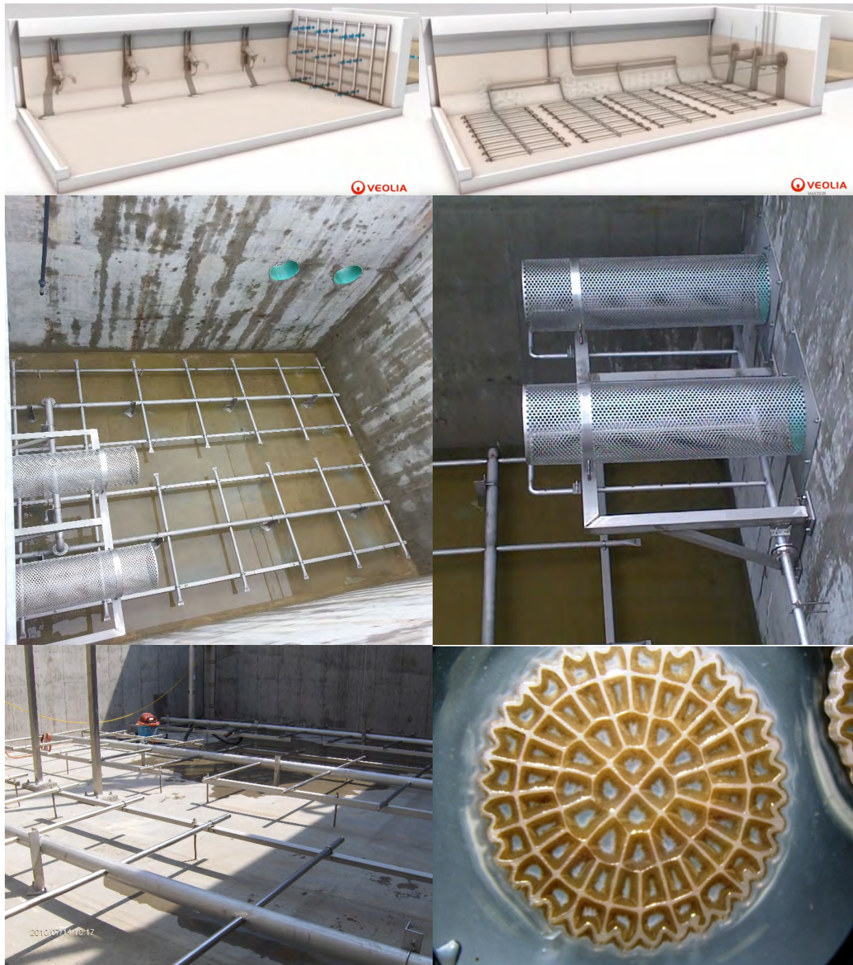
Figure 2-7 MBBR Components
