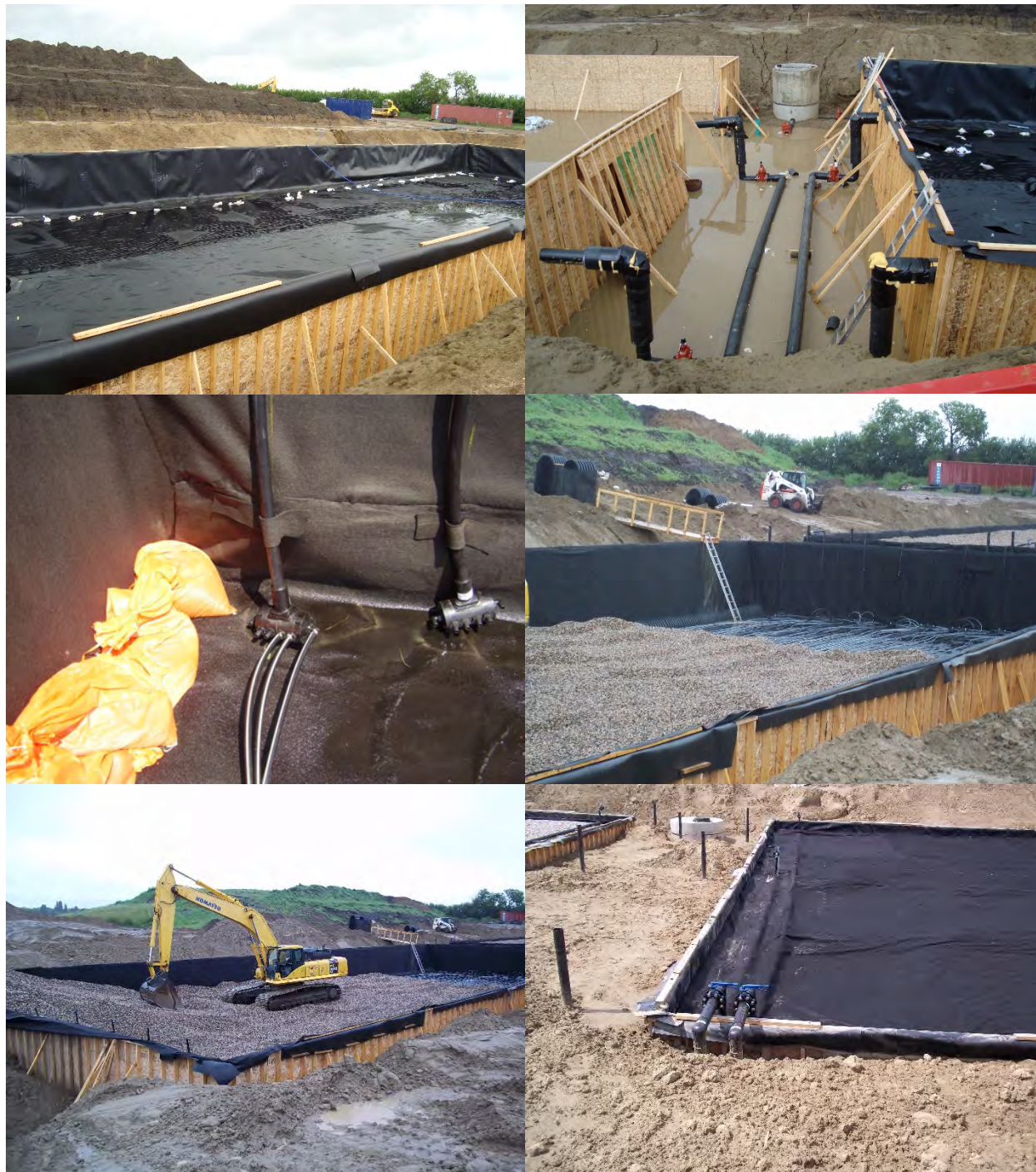
Figure 5-4 SAGR Components
