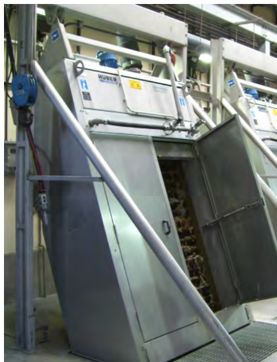
Figure 2-3 Step Screen
