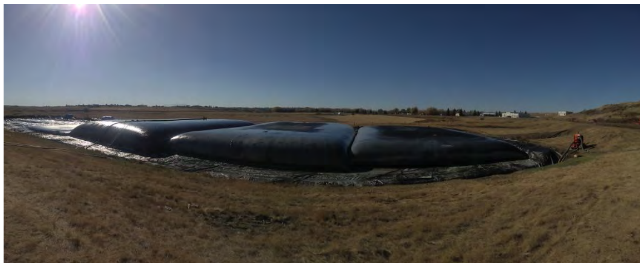
Figure 5-5 Lagoon De-sludging Using Geotextile Containers
