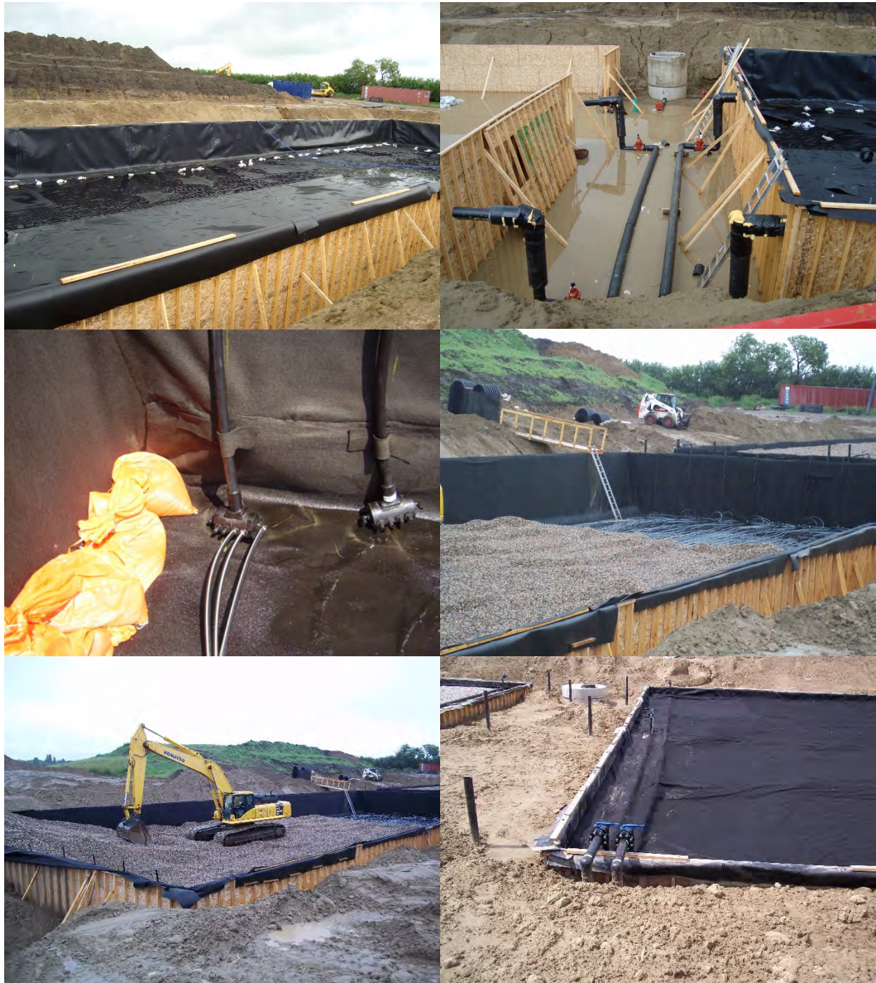
Figure 2-5 SAGR Components
