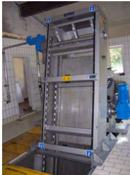
Figure 2-1 Multiple Rake Bar Screens
