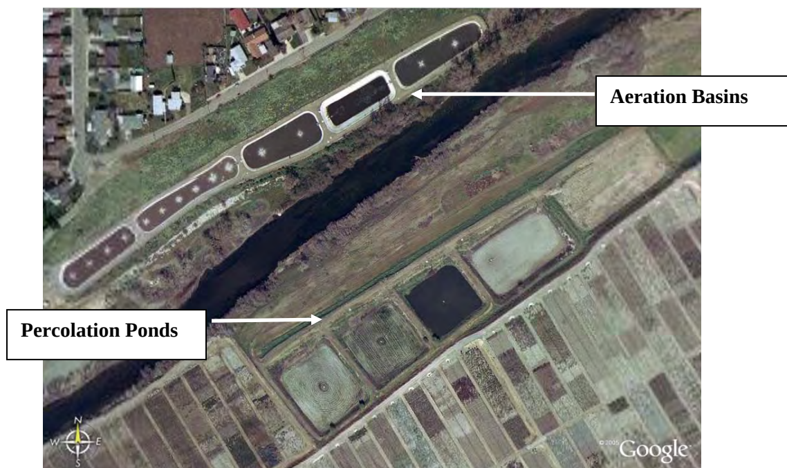
Figure 5 – Existing Waterford WWTP Site
