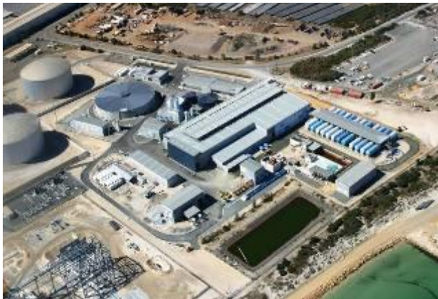
Perth Seawater Desalination Plant 2008
