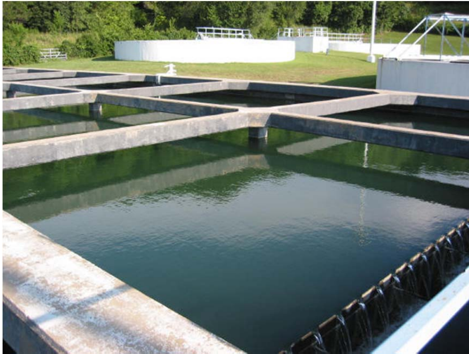
Top Photograph - Final Rectangle Sedimentation Basin Bottom - Clarifier
