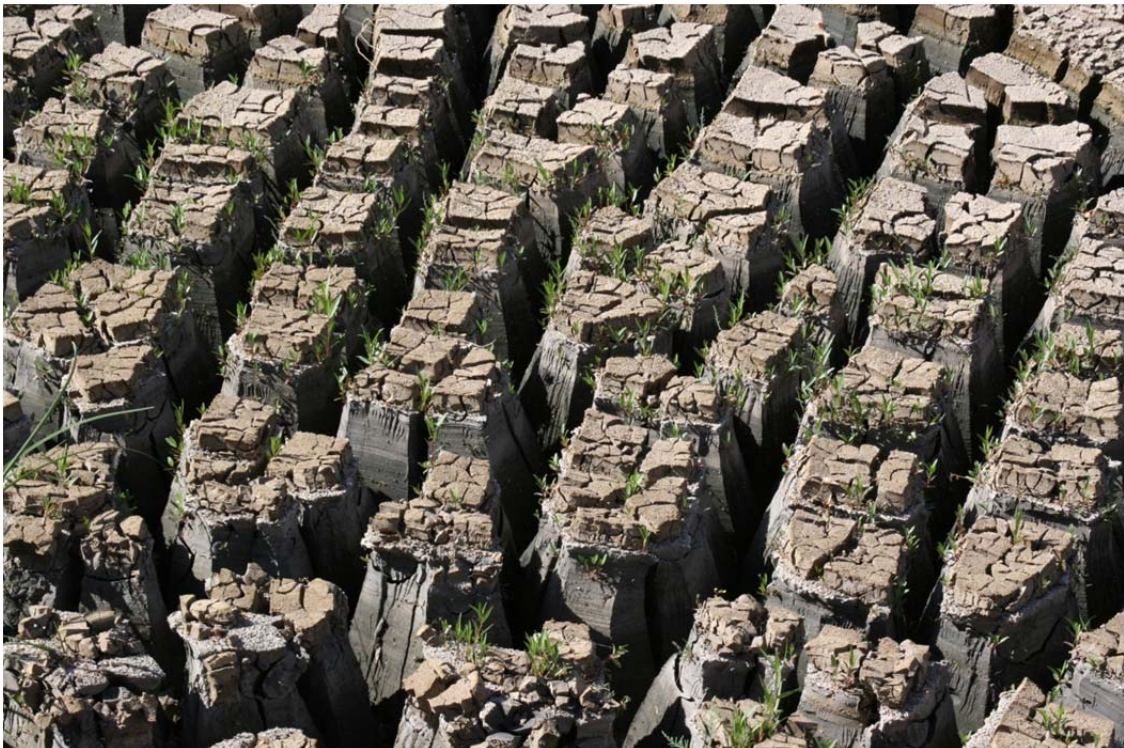
Pretreatment sedimentation basin, bottom photograph, sludge drying bed with new grass. Time to turn the sludge over.
