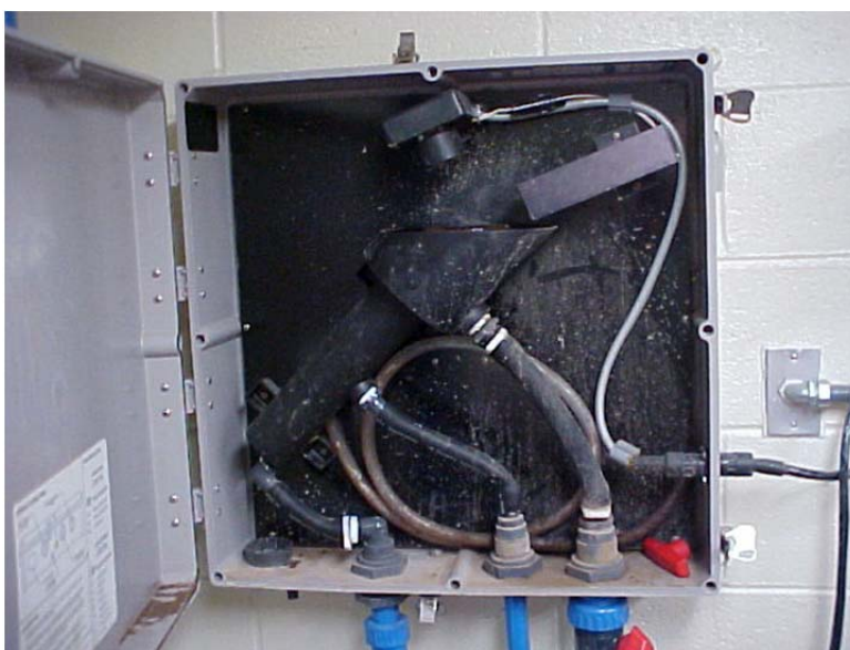
Inside a Turbimeter.
