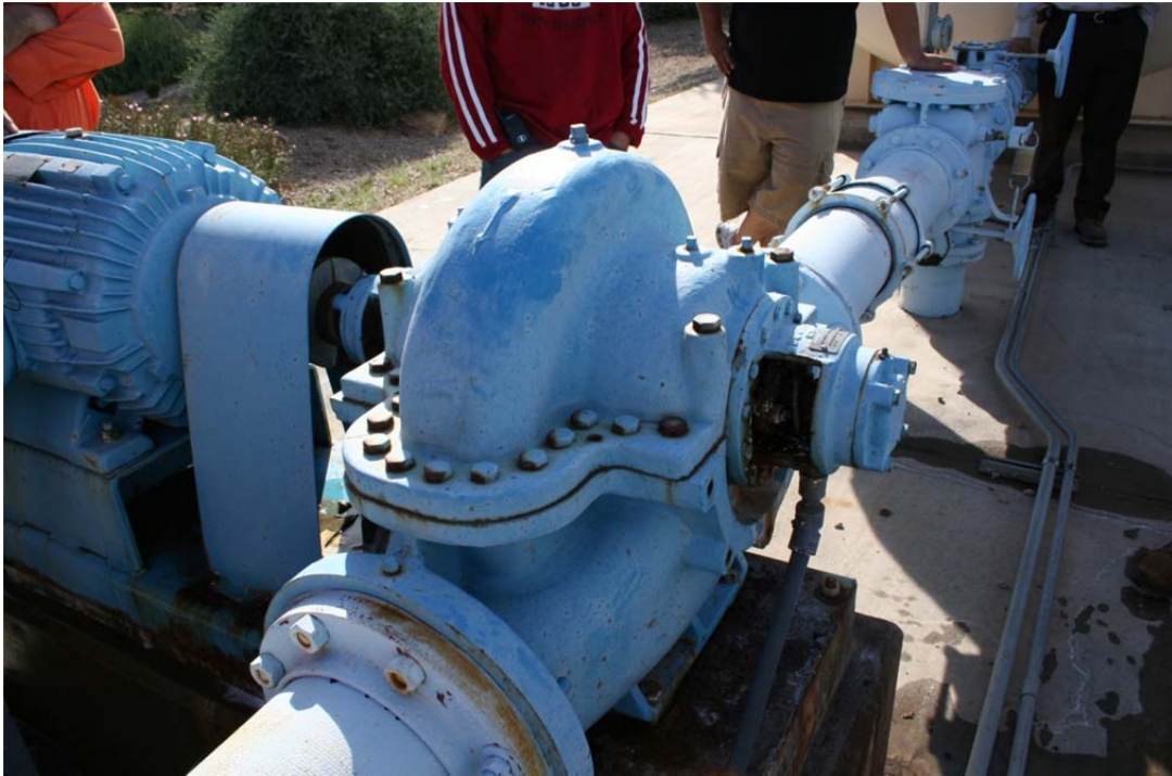
Split-case centrifugal pump.
