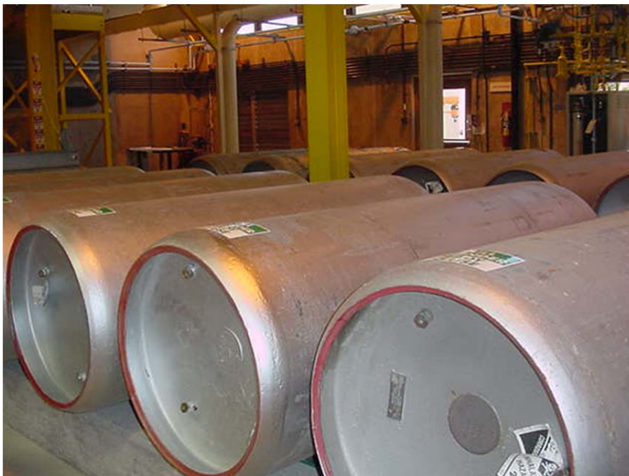
1-ton chlorine containers, rear side of container.
