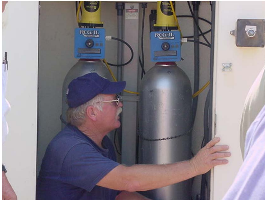
150-pound chlorine gas cylinder.
