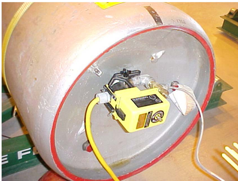
1-ton chlorine gas container with an automatic leak detection and shut-off device.
