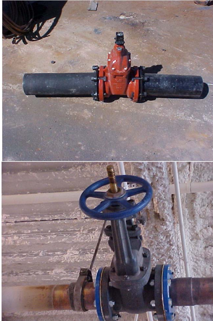
Different types of Gate Valves. (Linear)
