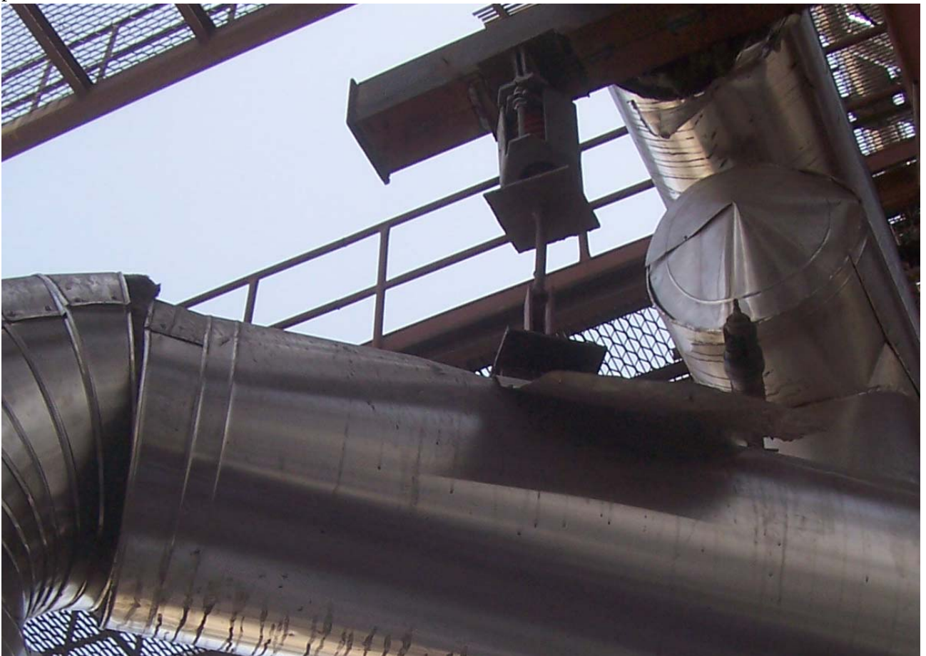
Photo 4: The Main steam line spring hanger is not carrying any load. The hanger rod from spring support is bent.
