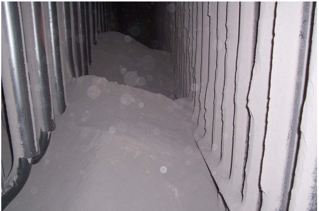
Photo 13: There is quite a good amount of ash accumulations seen in superheater area
