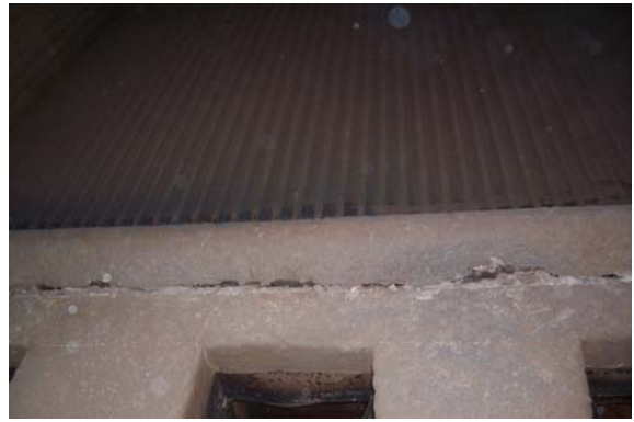
Photo 14: A clean furnace with bagasse as fuel.
