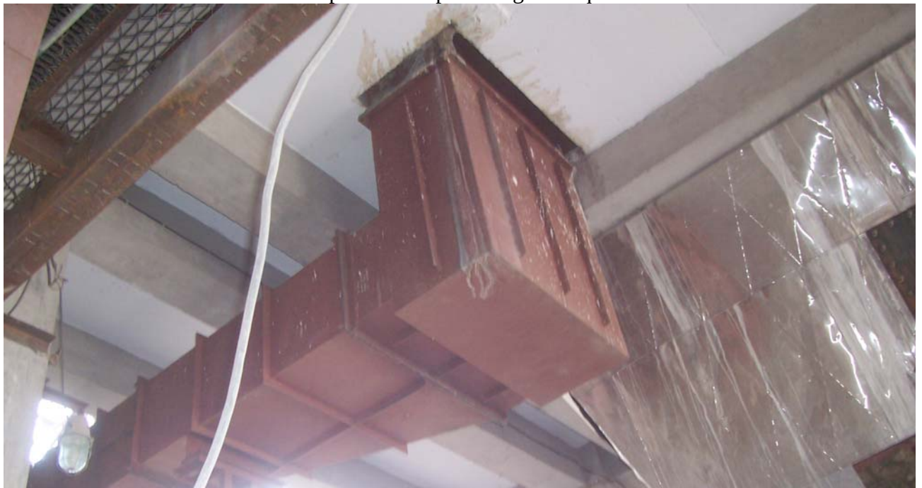
Photo 21. Today CFD has become a thrust area of energy conservation in terms of reducing unnecessary draft loss. But here, the PA duct bend is a right angle duct without a smooth bend.
