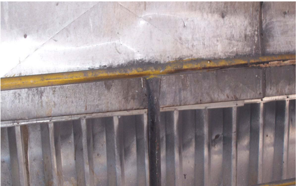
Case study 7 -Photo 14: dust leakage seen around the side cladding sheet below the penthouse.
