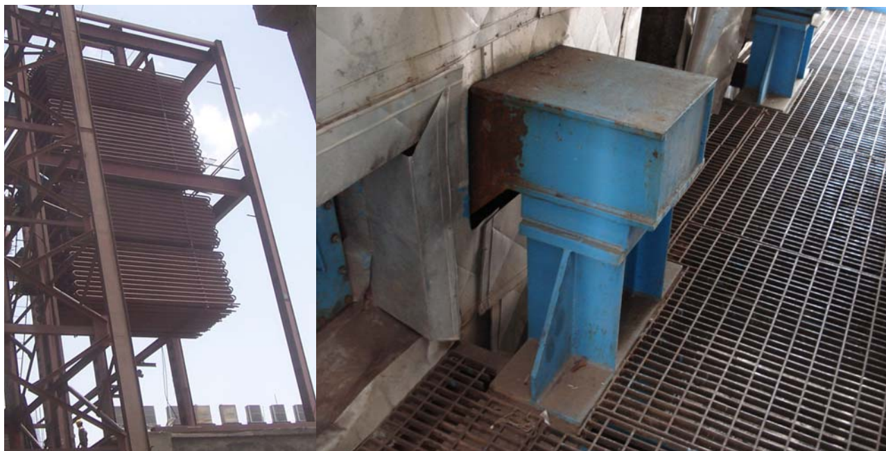
Photo 22 & 23: The economiser support beams are directly welded to support columns in this design. Other reputed manufacturers allow free thermal expansion of Economiser / APH as shown on the photo on right. The manufacturer needs to update their design.
