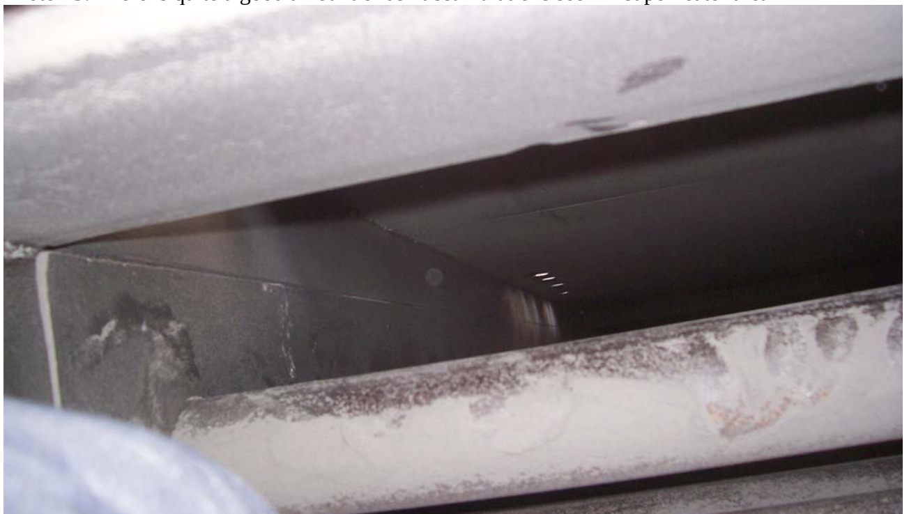
Photo14. The APH end tube to casing clearance is about 100 mm. Due to excessive gap the gas had bypassed and eroded the tube surface that is facing the casing.
