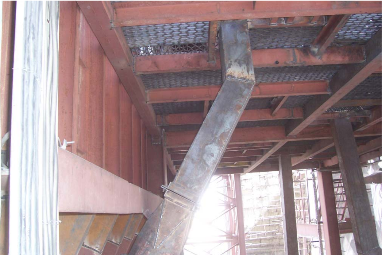
Photo 7: Limestone feed chute is of rectangular. This would give problem as the limestone is hygroscopic. The Limestone has to be connected to drag chain feeder directly.
