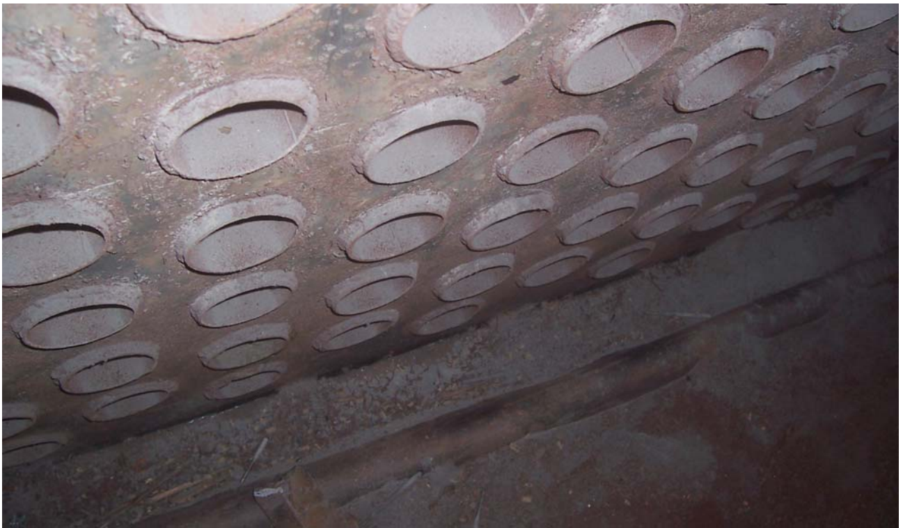
Photo 21: APH outlet duct is only stitch welded at erection stage itself. The field quality inspection system is missing. The hot air is leaking to outside.
