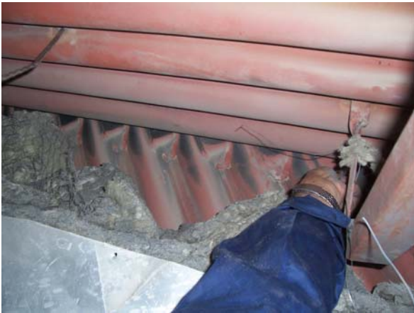
Photo 7: Indications of dust below waterwall nose panel. The seal was not done as per drawing.
