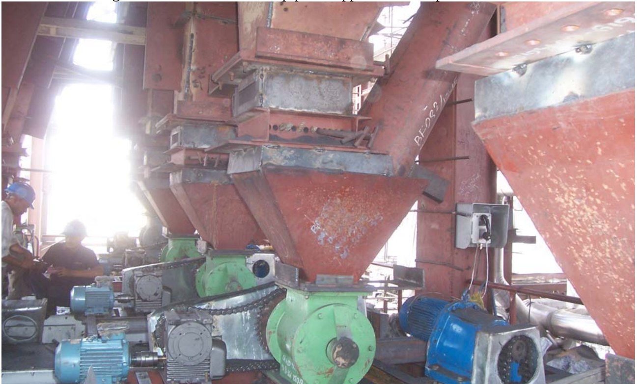
Photo 6: Already the feeder is of under capacity for petcoke. To this feeder, the limestone chute is connected. Moreover the petcoke regulation is not possible when limestone mixing is done like this. This is a very fundamental mistake.
