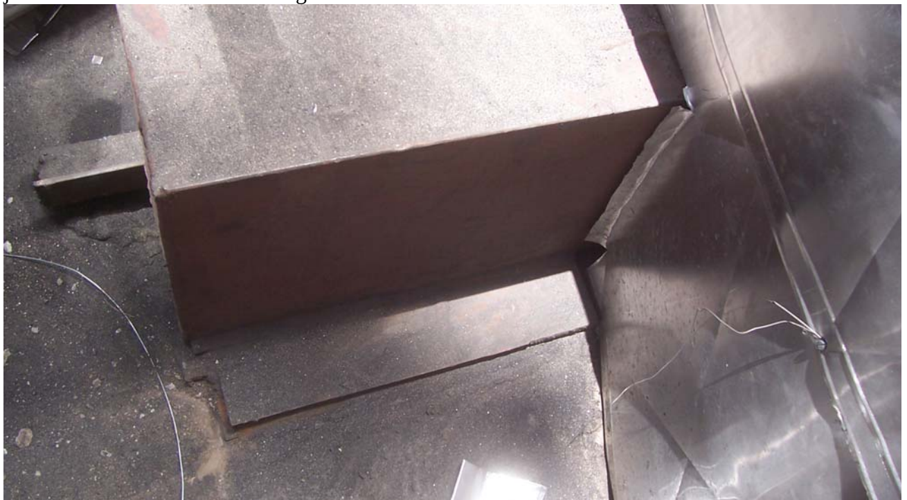
Photo16. All the APH base supports are directly welded to insert plates on the RCC. This restricts the thermal expansion and this RCC may damage.
