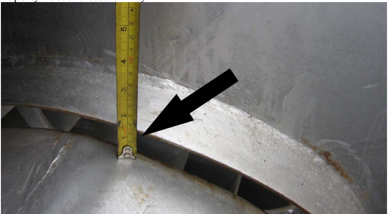
Photo 2: The impeller to suction casing clearance is around 30 mm all around. This can cause recirculation of flue gas. Thus the draft will be less at furnace.
