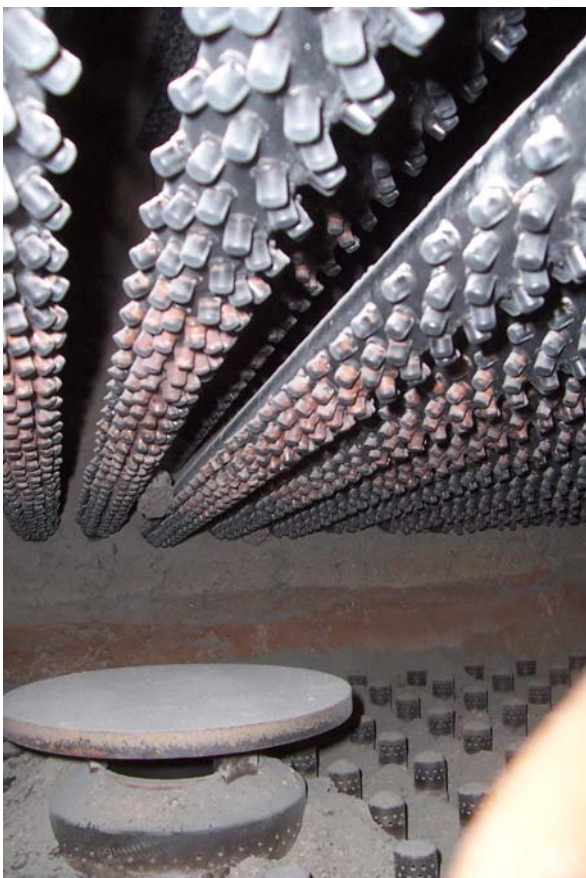
Photo 1-3: Photos above illustrate the ash fouling above coal nozzles. Blunting of outer studs is seen.
