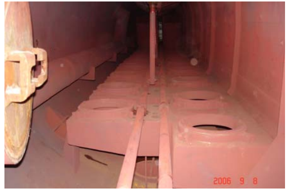
Photo 2: Chemical dosing line is laid closer to blow down line. Cyclones dismantled.
