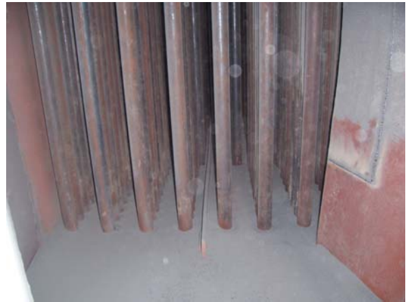
Photo 8: Ash inside airpreheater confirms failure of preheater tubes. FD air directly mixing with flue gas can lead to starvation inside furnace.
