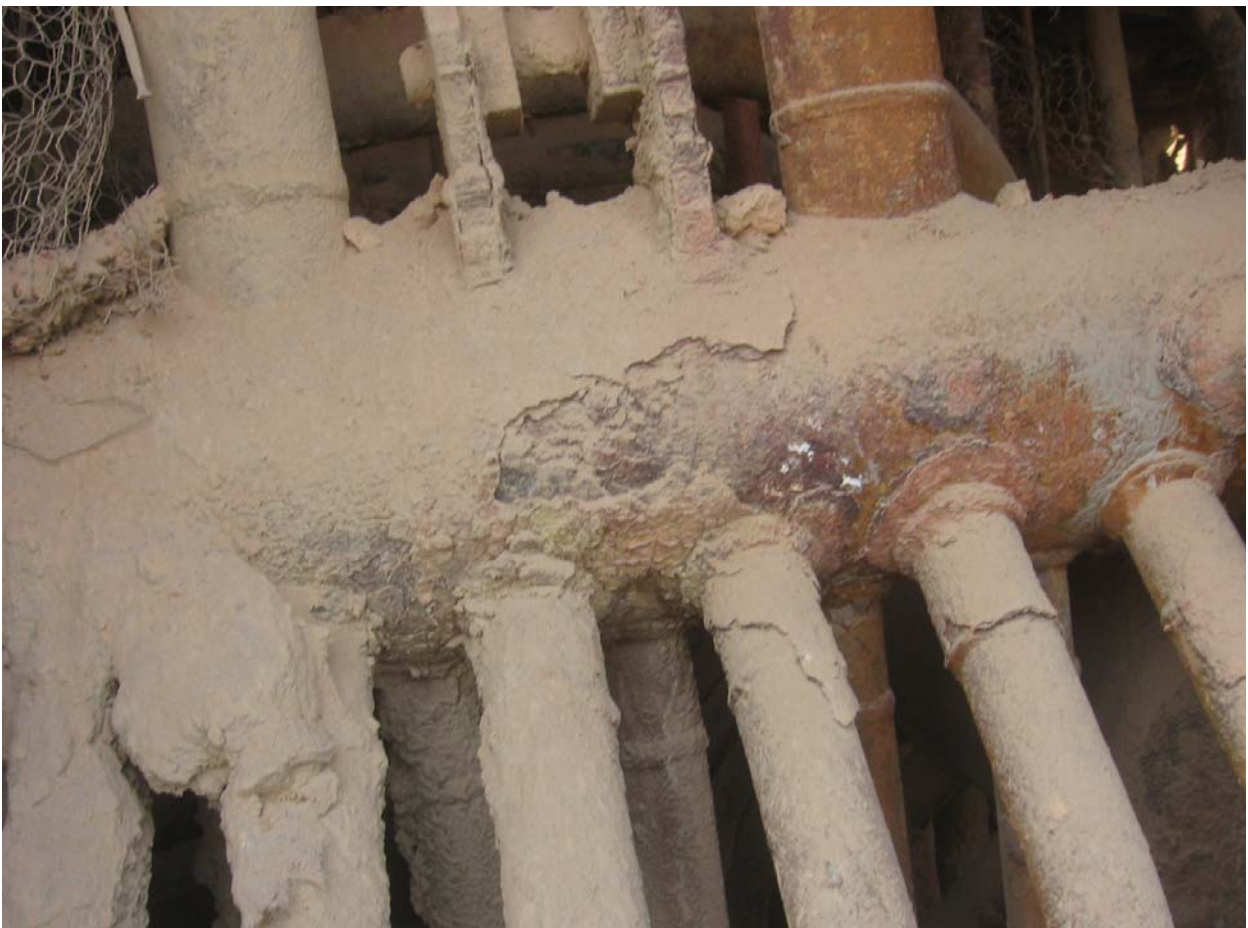
Case study 2: Photo 4: Corroded waterwall header due to condensation of flue gas.
