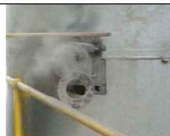
Photo 2: Backing of ash in the next loop seal.
