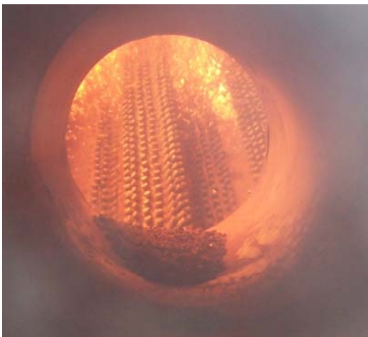
Photo 5-Improper fluidization –High DP drop
