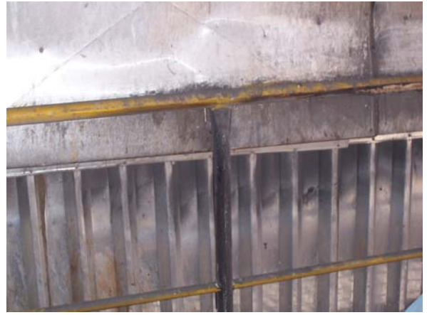
Photo 6: Indications of smoke at penthouse confirm air ingress. When the furnace pressure goes positive at times, the flue gas comes out.
