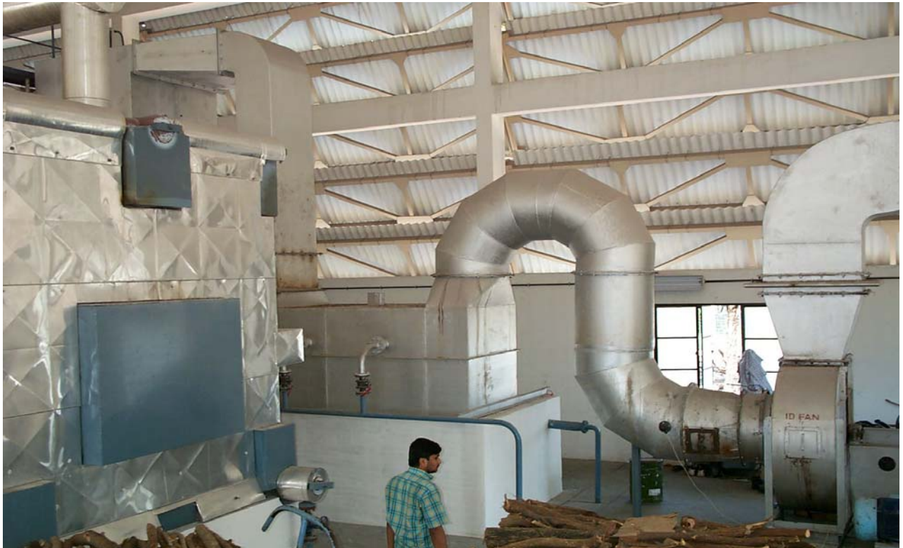
PHOTO 4: PHOTOGRAPH SHOWING THE WET BOTTOM DUST TRAP
