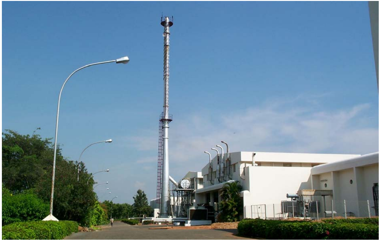
PHOTO 1: EXISTING OIL FIRED BOILER
