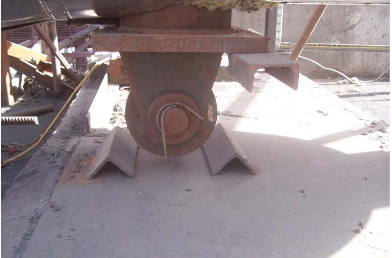
Photo 25: Boiler thermal expansion guide is not strong enough. This needs redesign.
