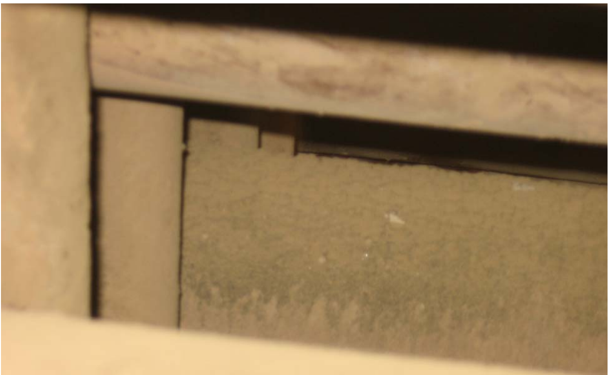
Case study 7- Photo 16: Flue gas condensation as droplets over the ash is seen. A proof air ingress & ash leak.
