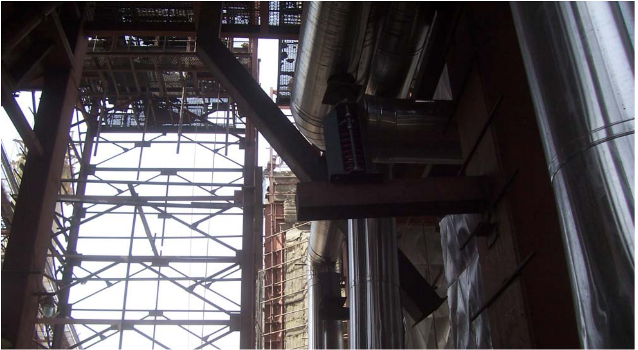
Photo 3: The Spring support base is distorted / erected improperly. A bracket could have been provided.
