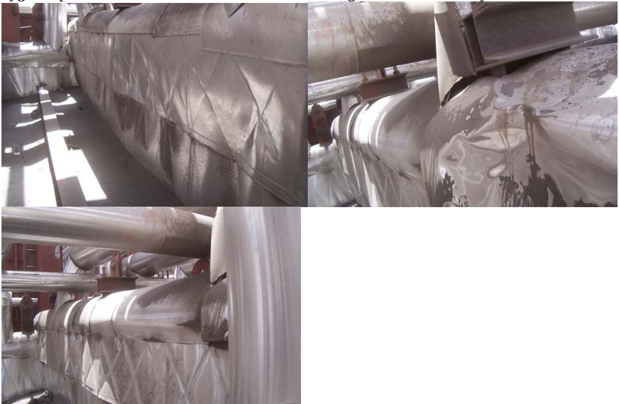
Photo 8,9 &10: Roof panel to CSH / RSH sealing is not OK. Ash is seen in the insulation cladding. Oxygen can not be taken as a guide for setting the air flow, since the air ingress will mislead.
