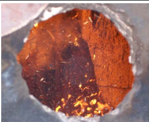
Photo 17: Poor fluidization in furnace - mal-operation
