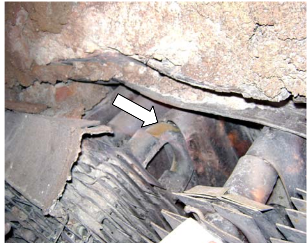
Case 6: The protection shield at bends was not placed properly during maintenance. This had led to a stoppage of the plant. There is a gas baffle to prevent the gas going along the bends.
