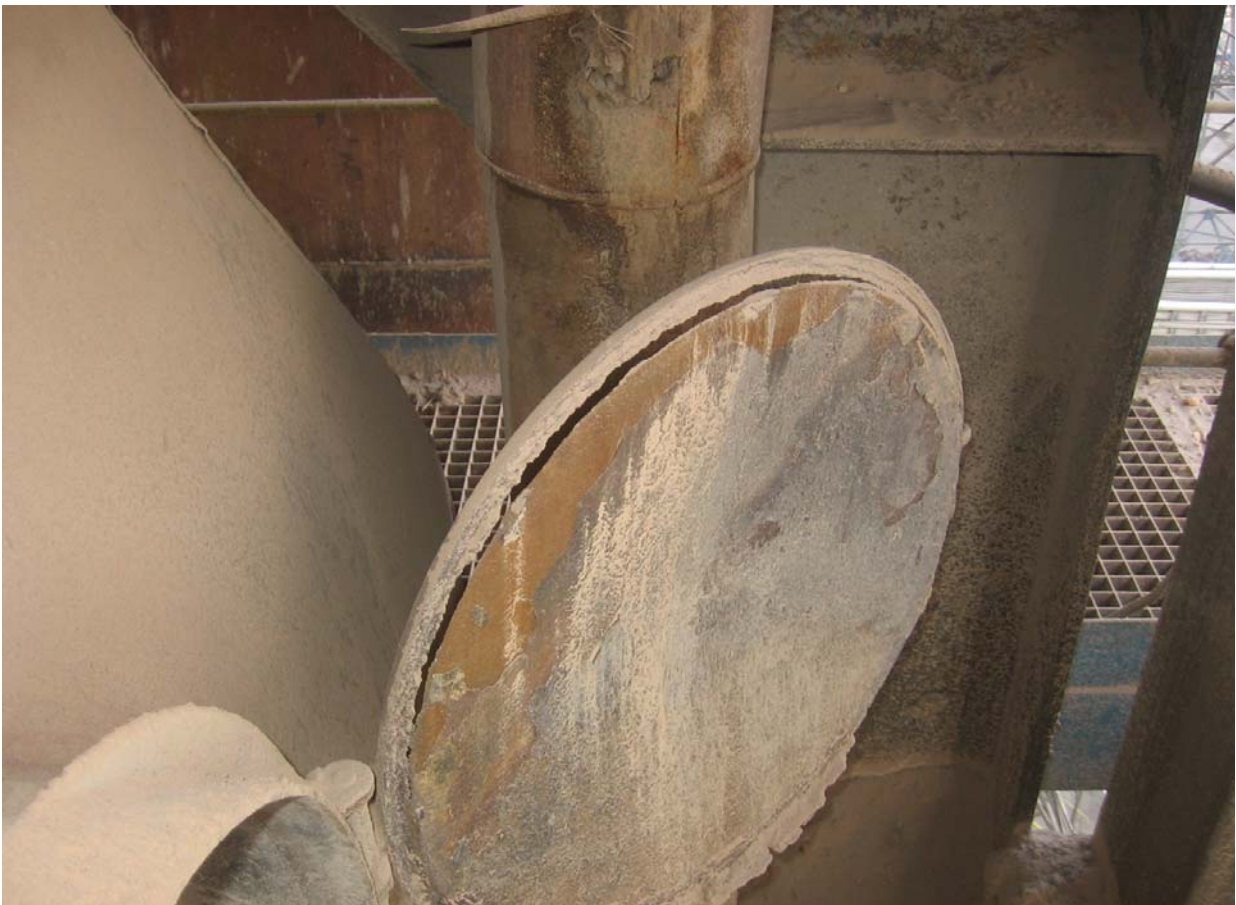
Case study 2: Photo 6: leaky penthouse door.
