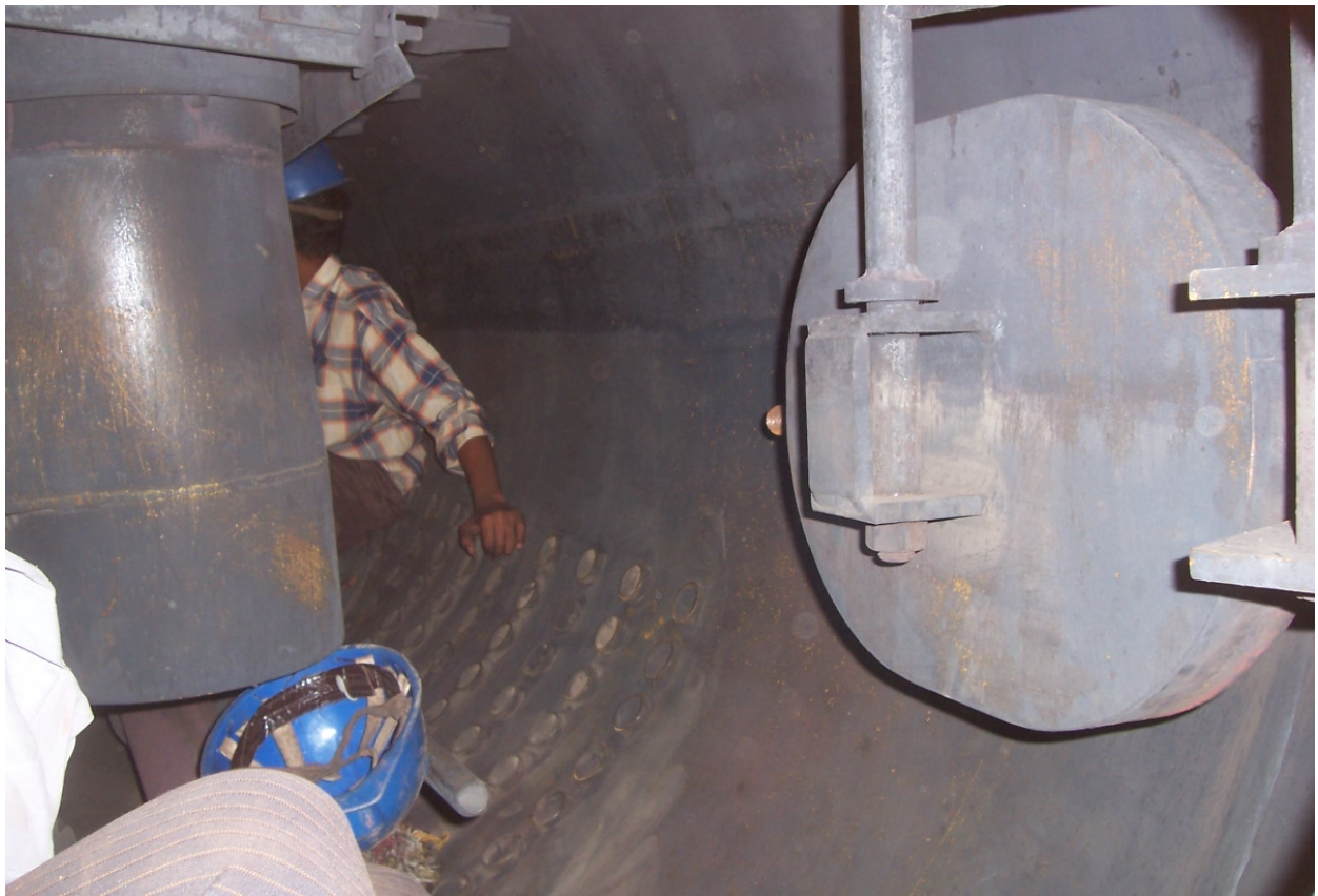
Photo 11: This is a boiler wherein the drum internal surface & turbo separators indicate the perfect boiler water chemistry.
