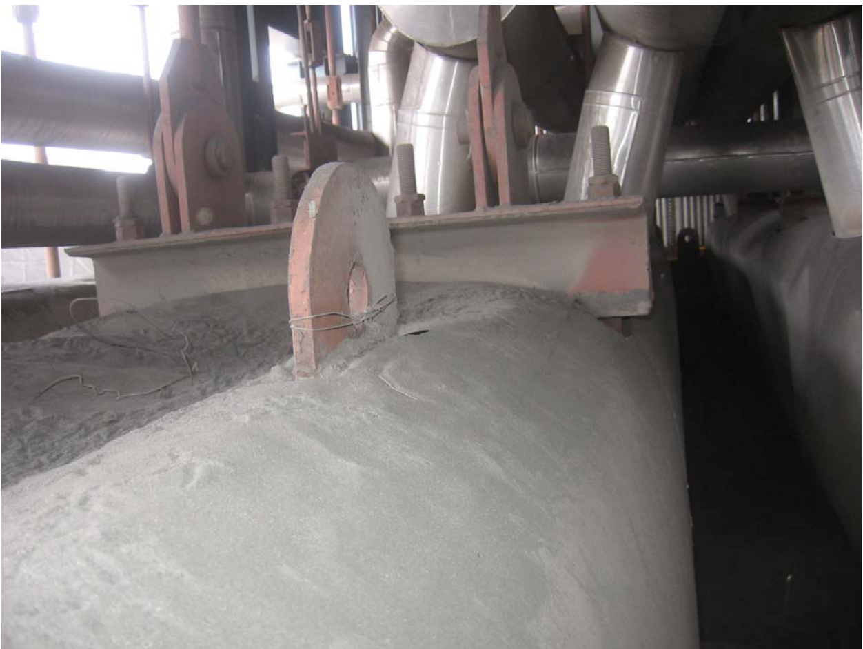
Case study 6- Photo 13- Ash leakage marks at SH header area above the roof in a new boiler.
