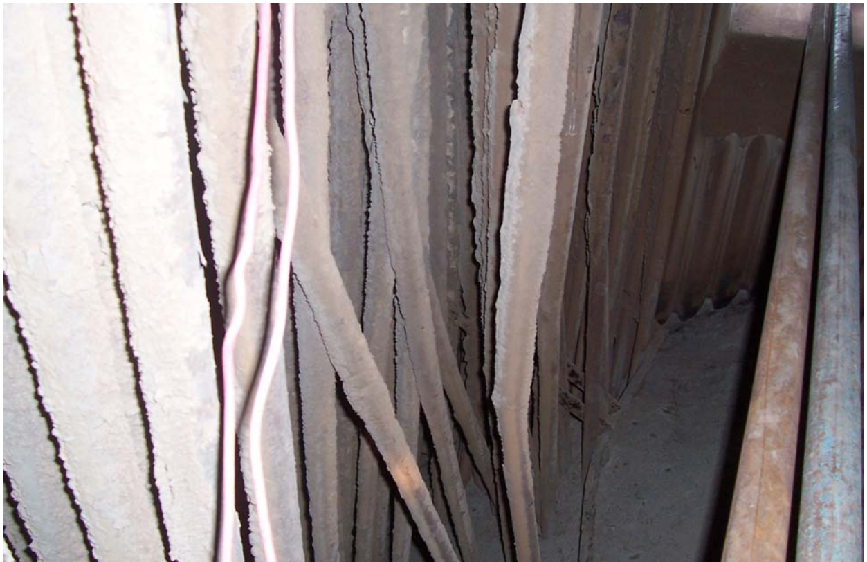
Case study 1 : Photo 1- The Superheater coils distorted due to spacer / support clamp corrosion failure.
