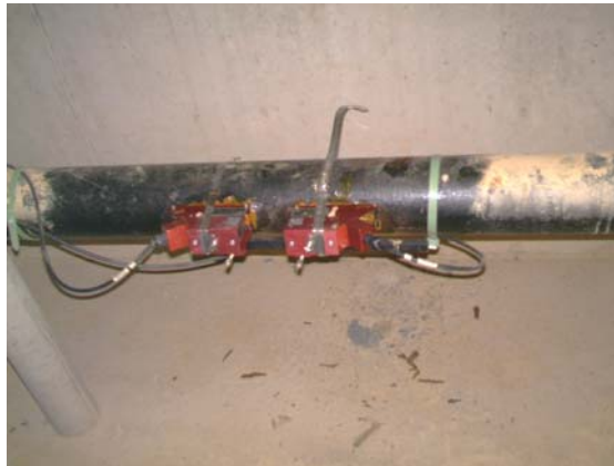
Figure 2.22 – Ultrasonic strap on meter
