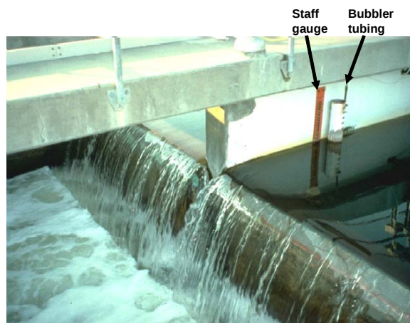
Figure 5.6 – Staff gauge as a backup to a bubbler system 6
