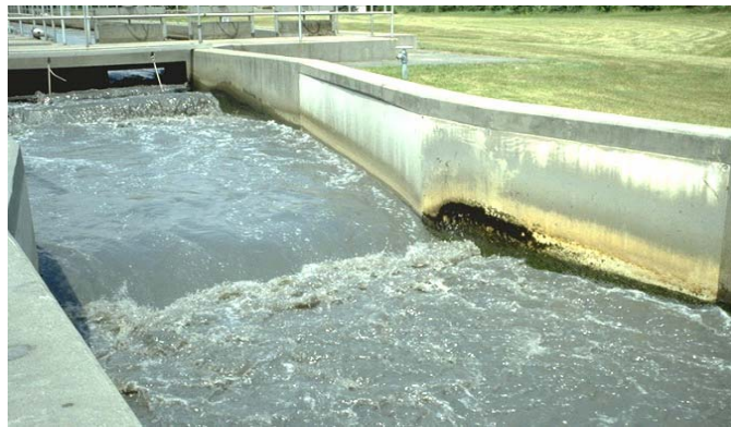
Figure 5.1 – Beginning Stages of a Submerged Condition 1
