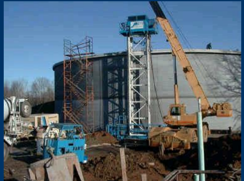
Prestressed concrete water storage reservoir
