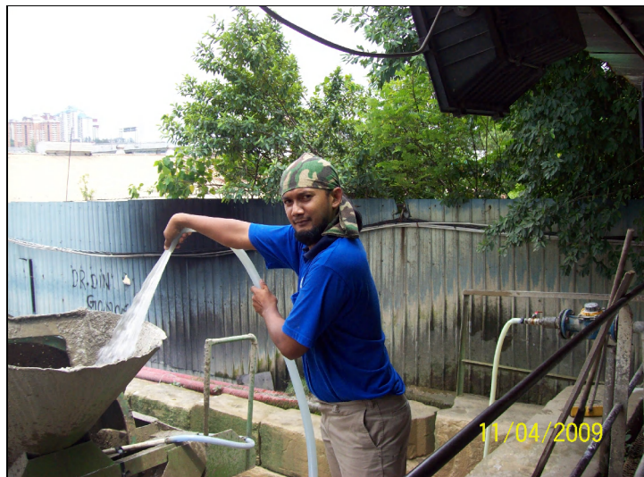
Figure 3.4 : Treated waste water is mixing in the concrete truck mix drum.
