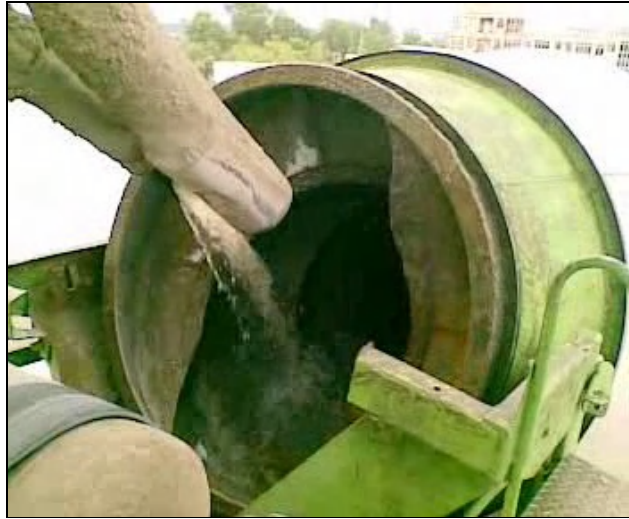
Figure 3.3 : Potable water mixed in the concrete truck mixer drum
