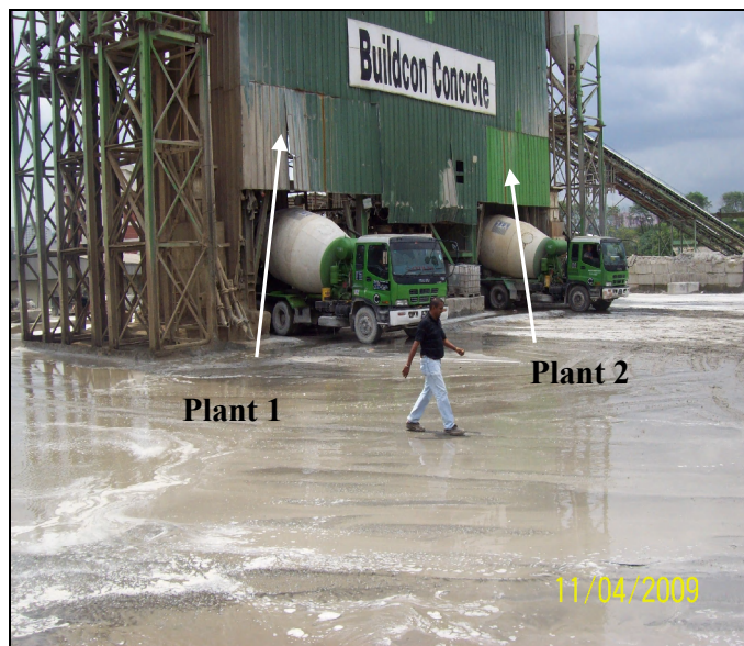
Figure 3.2: Plant 1 and Plant 2 ( Wet mix )
