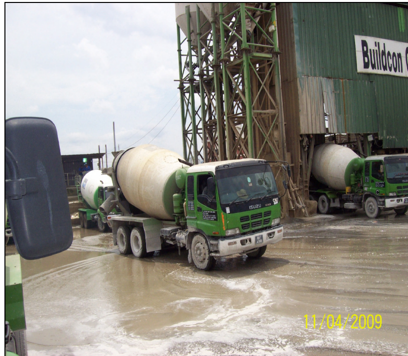
Figure 1.2 : Concrete batching plant
