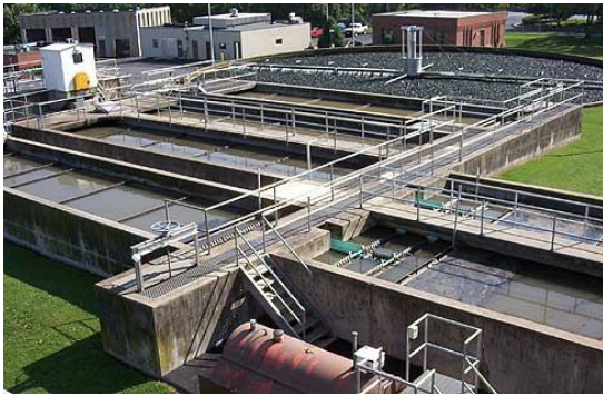
Typical View of Primary Clarifier
