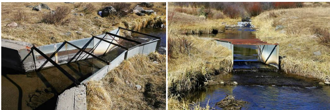
Fig 3.2 Parshall flume in operation
