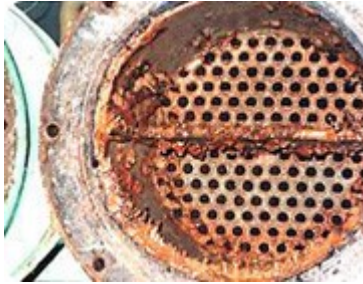
Tubes just after manual cleaning
