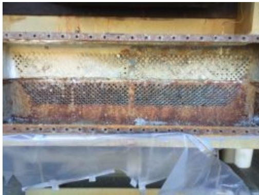
Severe scale-calcium buildup on a Trane Absorber
