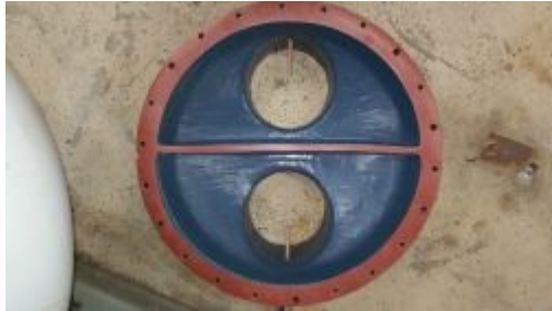
Finished Belzona Epoxy Coating on Tubesheet
