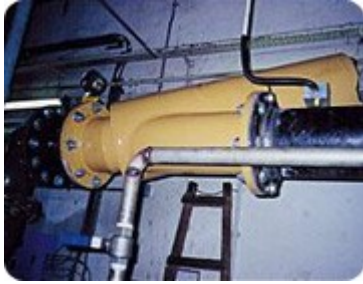
Tubes before cleaning
