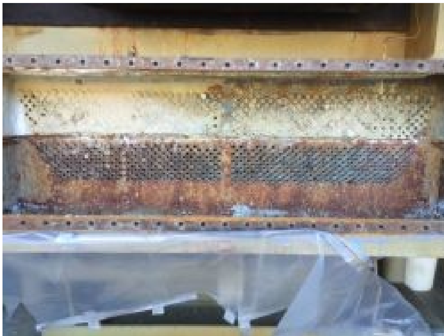
Severe scale-calcium buildup on a Trane Absorber
