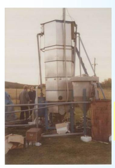
The first pilot trial on Tertiary filtration of municipal waste water was carried out in August 1978.
