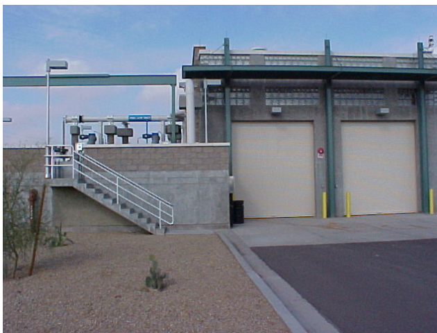
Wastewater Treatment Headworks
