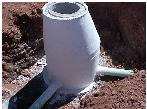
Newly finished Manhole and Laterals.
