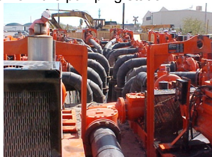
Pumps at a temporary sewer manhole by-pass.
