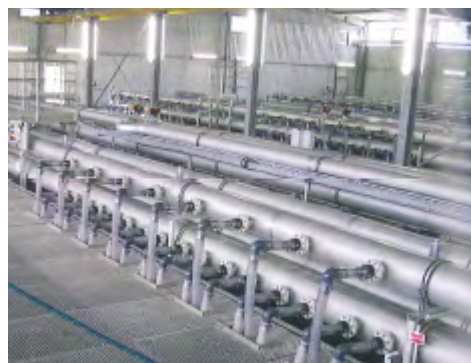
Figure 8.5 membrane installation at the WWTP Nordkanal
