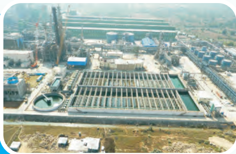
Effluent treatment plant at a steel industry
