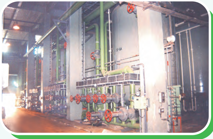
Softener at a power plant
