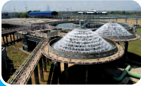
Cascade aeration at a power plant
