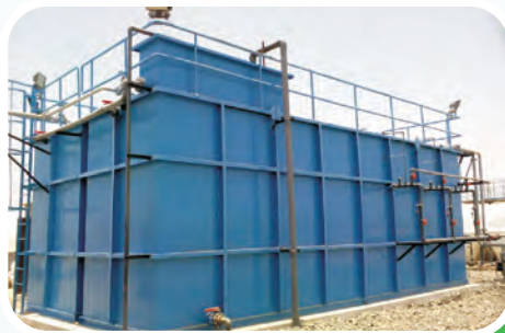
Membrane bioreactor at a construction company
