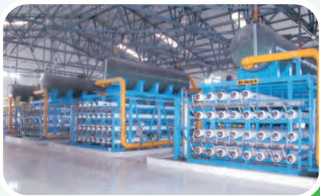
Sea water reverse osmosis at a power plant
