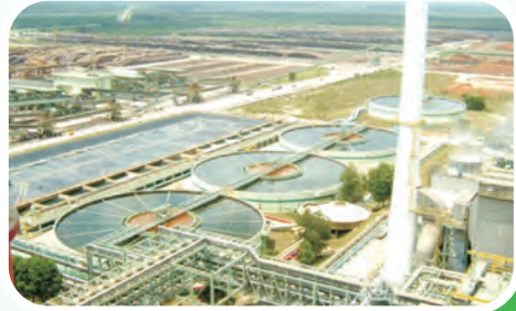
Clarifiers section at a paper plant
