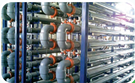
Membrane application at an automotive industry
