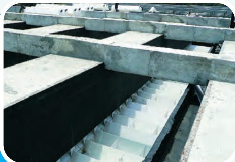
Upflow anaerobic sludge blanket (UASB) at a paper industry
