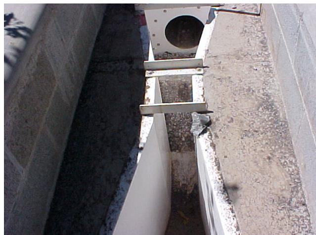
Parshall Flume and Ultrasonic Flow Meter. Here is a great trick if you do not have a stand for your ultrasonic probe, simply use a reflective street cone to hold your probe. Notice the debris and most POTW's will write a NOV for not maintaining the flume and/or uncleanness.
