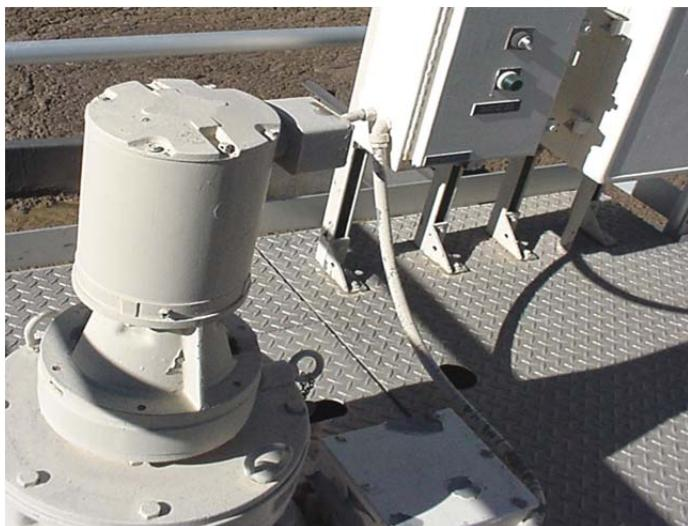
Most vertical motors are mounted on a gear reduction unit as seen in the photograph on the right. The impeller drive shaft can be enclosed in a housing connected directly to the gear box. There is a bearing at the bottom of the shaft that steadies and aligns this shaft. This bearing needs lubrication, always check your manufacturer's recommendations.
