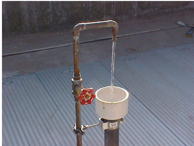
Water Sample Station commonly found at most water or wastewater treatment plants. This tap will allow the operator to obtain Grab Samples for pH, Temperature, COD, Bacterial, ORP, OUP, Organics and Inorganic field parameters.
