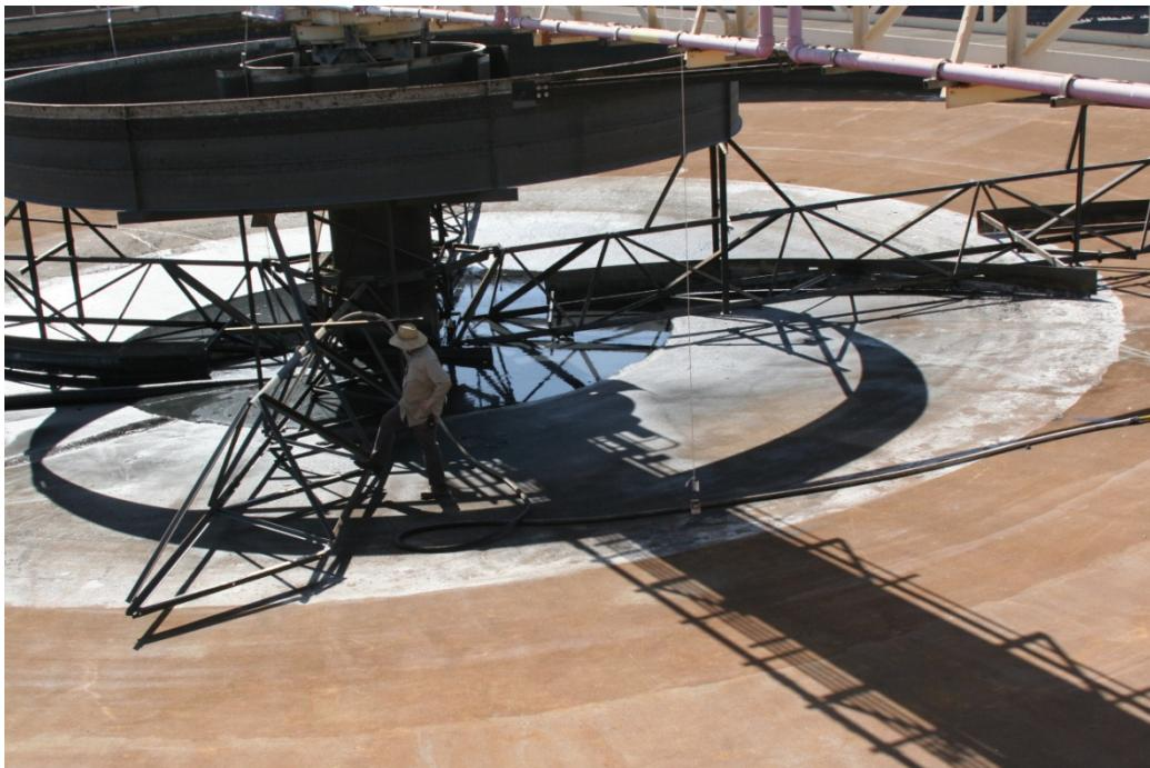
Scraping mechanism inside a clarifier.
