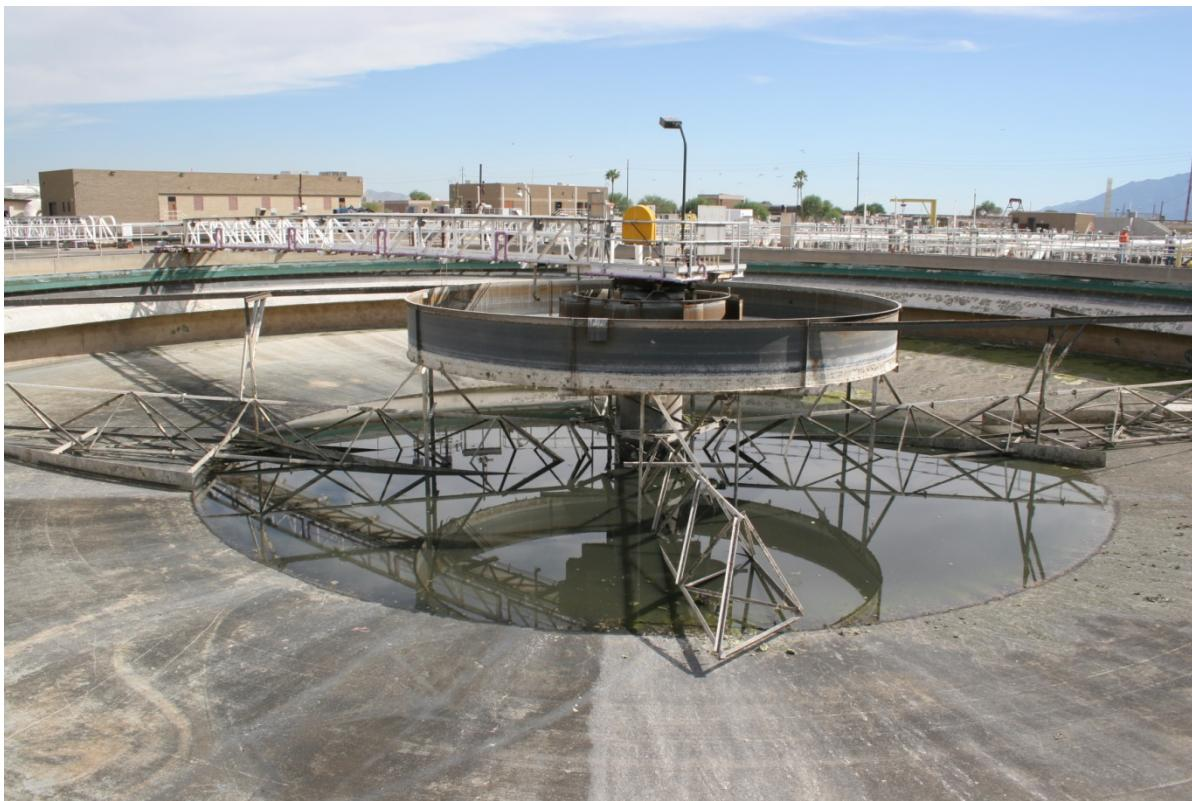
Top photograph, a clarifier's raking mechanism.
