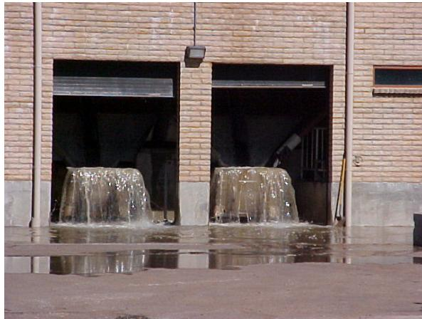
Domestic waste overflow at the head works. Yes, incredibly headworks do overflow, usually due to rags, grease and debris or operator error. We do not like to see this happening and are very careful about letting the public and state regulatory agencies see this activity. One activity the State does not want to see but will happen during a rain storm is bypassing untreated waste to the outfall.
