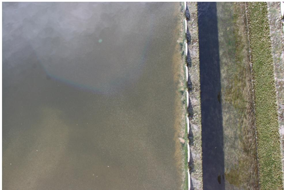
Here is Pen floc being carried over the weir do to a process upset. Algae growth in excess can also create several different problems.
