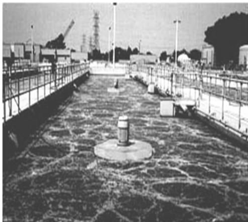
The motor speeds are usually in the 1800 rpm range. This speed is reduced to the 30 to 70 rpm range with gear reducers.
