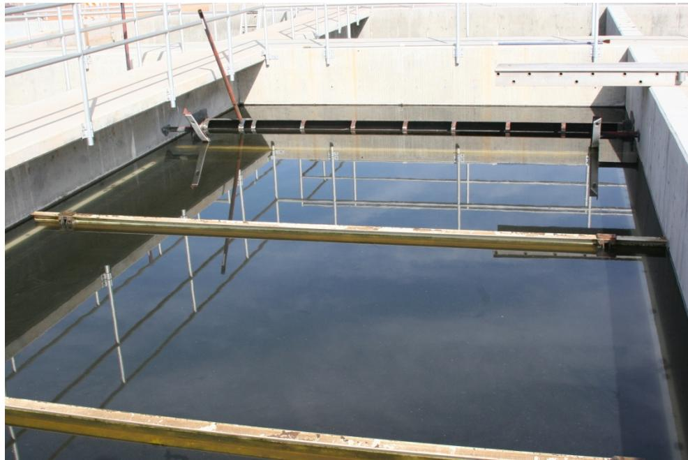
Here is an example of a rectangular clarifier used in the secondary settling process. Operation changes that should be employed if a dark brown foam is developing on the aeration basin is to increase the wasting rate.
