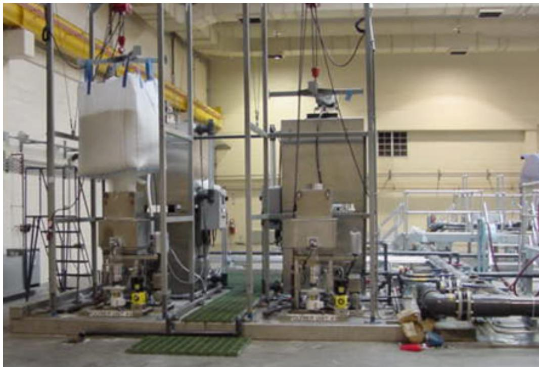
Dry polymer is being added and used for sludge thickening.
