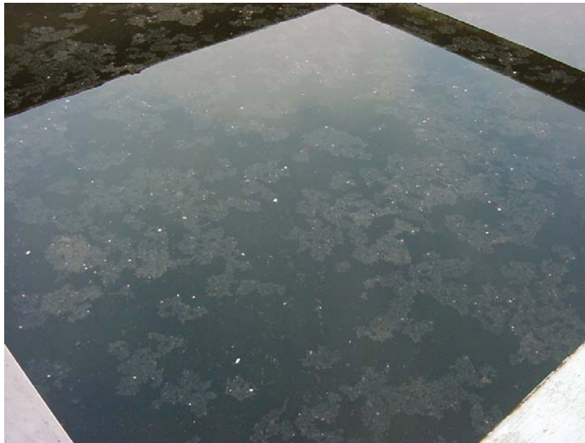
Figure 8: Ashing on clarifier surface
