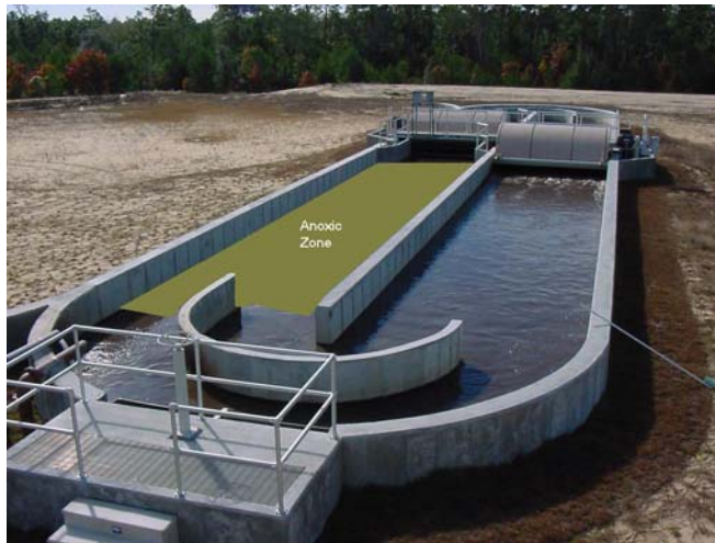
Cover Photo: Oxidation ditch WWTP with anoxic area highlighted
