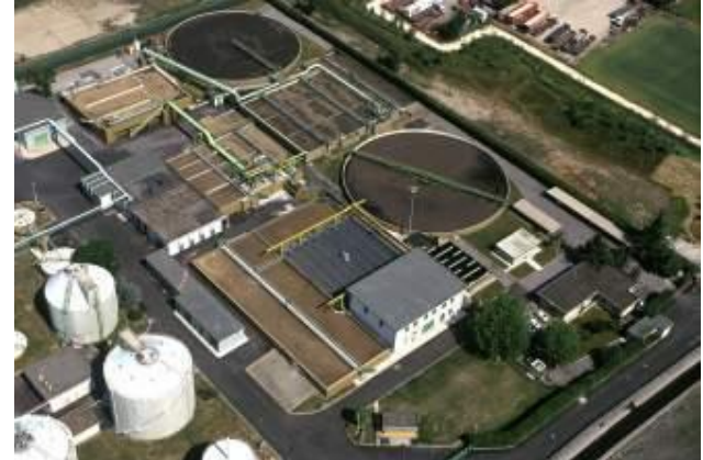
Brescia, Italy: Membranes retrofit into existing activated sludge treatment lines
