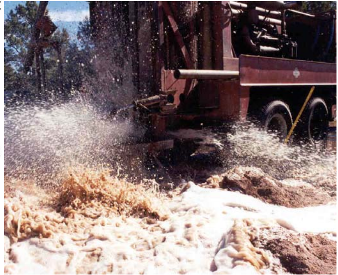
Surge of Air Developing a Well.
