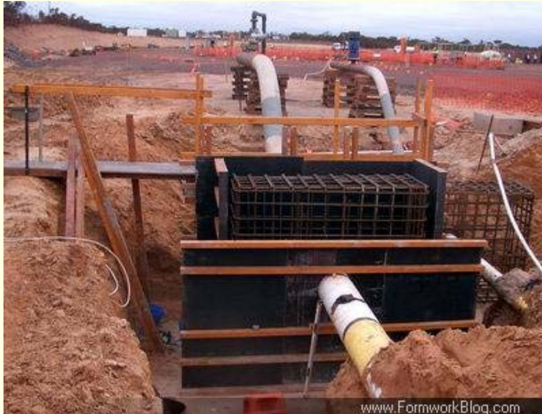
Fig. 5.33 Thrust block under construction
