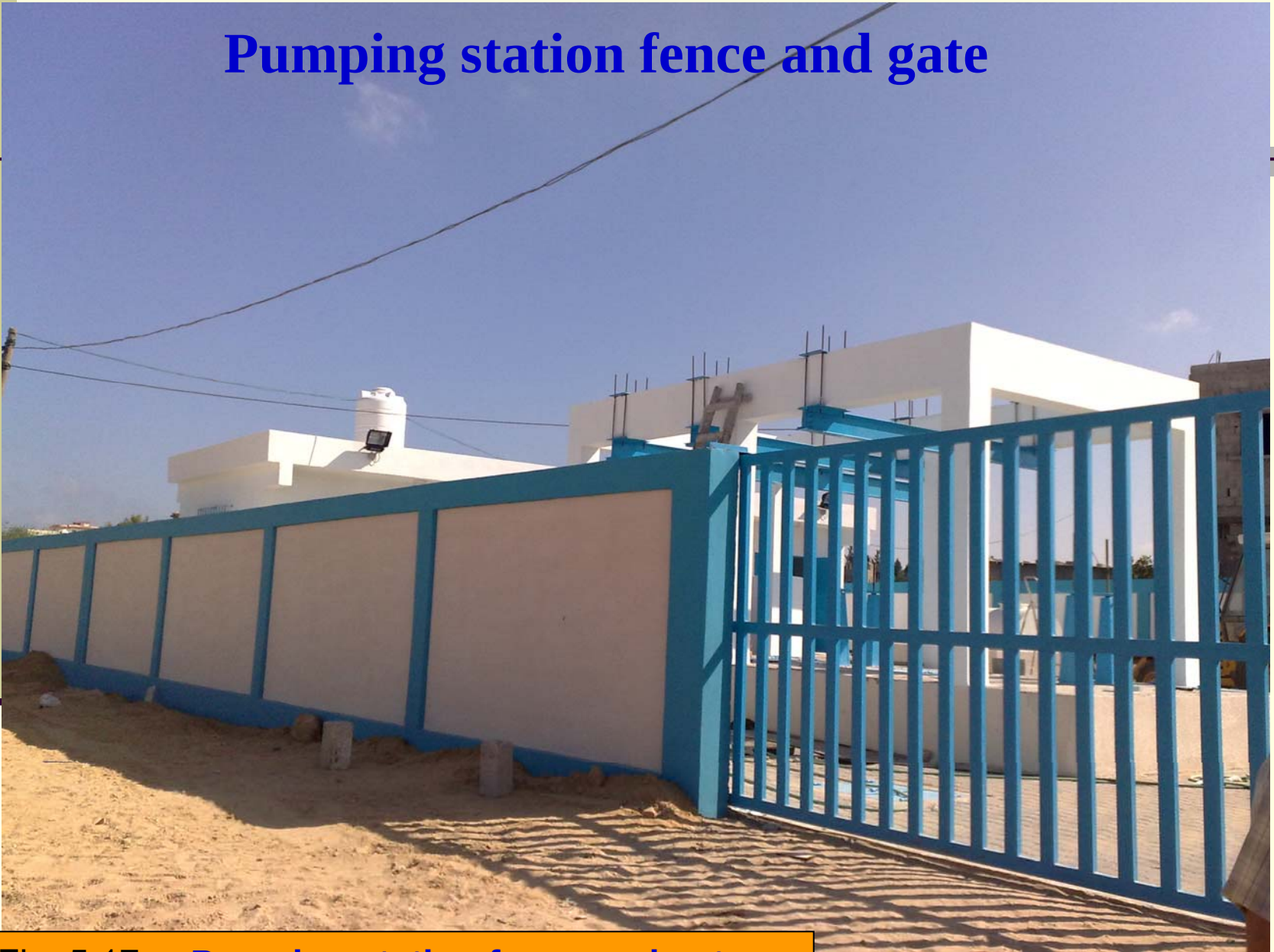
Fig. 5.17 Pumping station fence and gate
