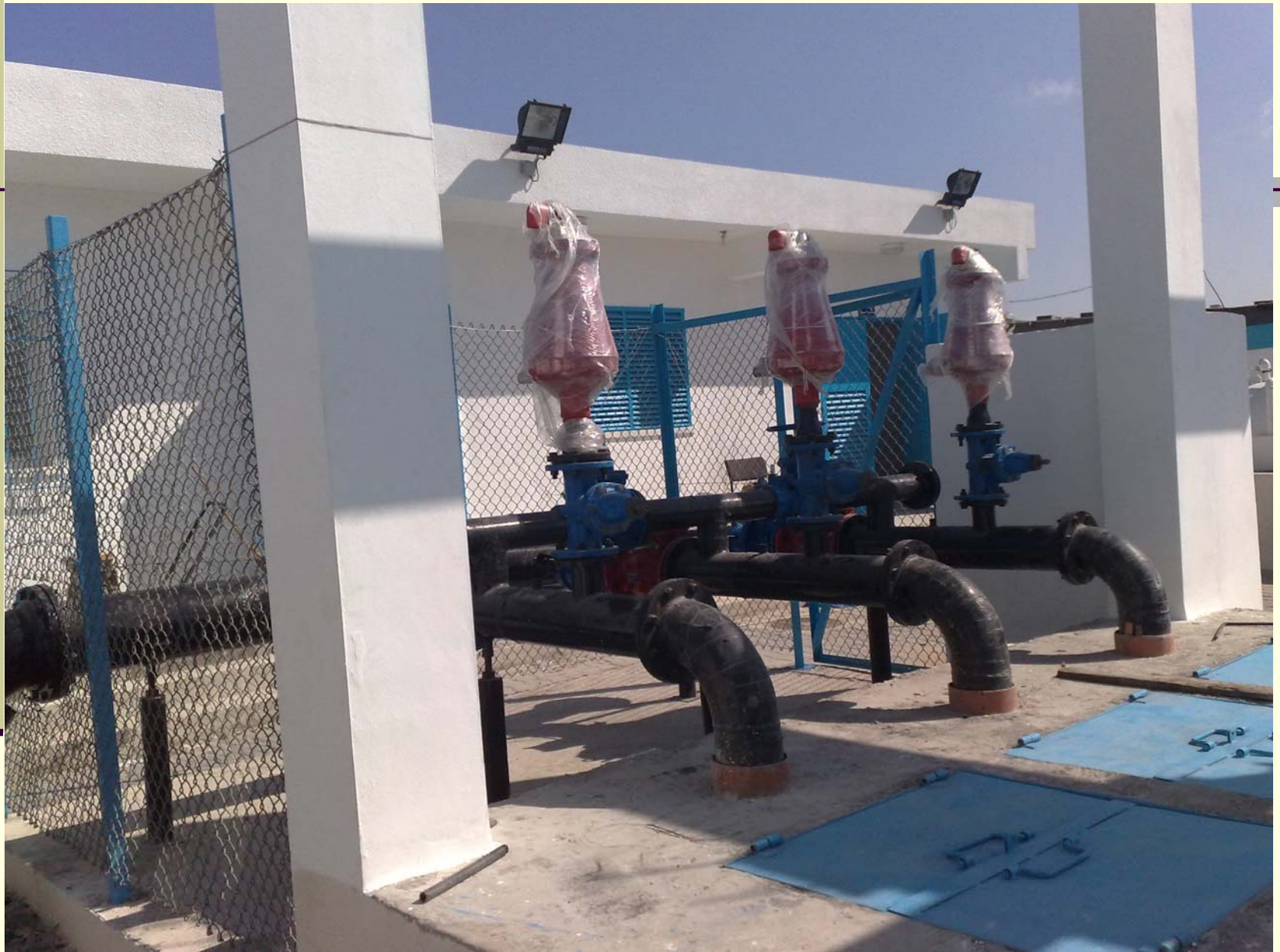
Fig. 5.27 A photo at the top of a wet well showing delivery pipes and valves
