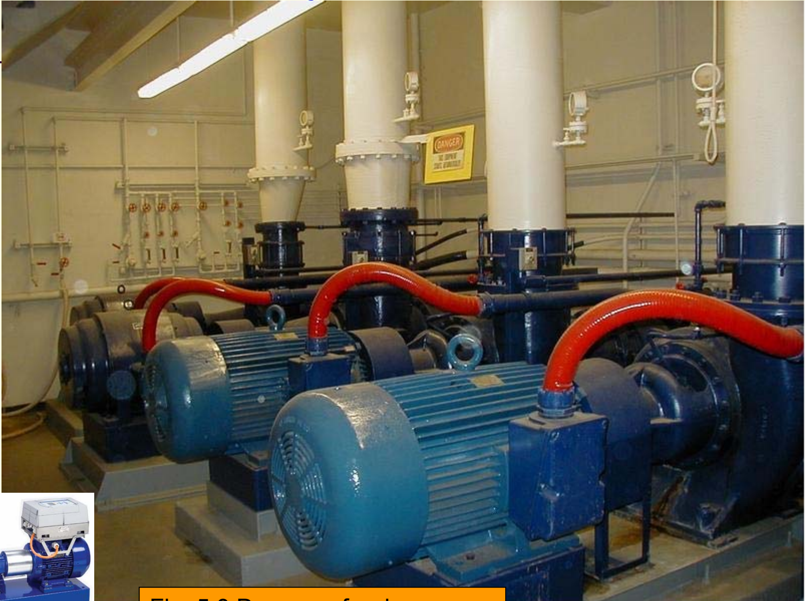
Fig. 5.8 Dry room for dry pumps
