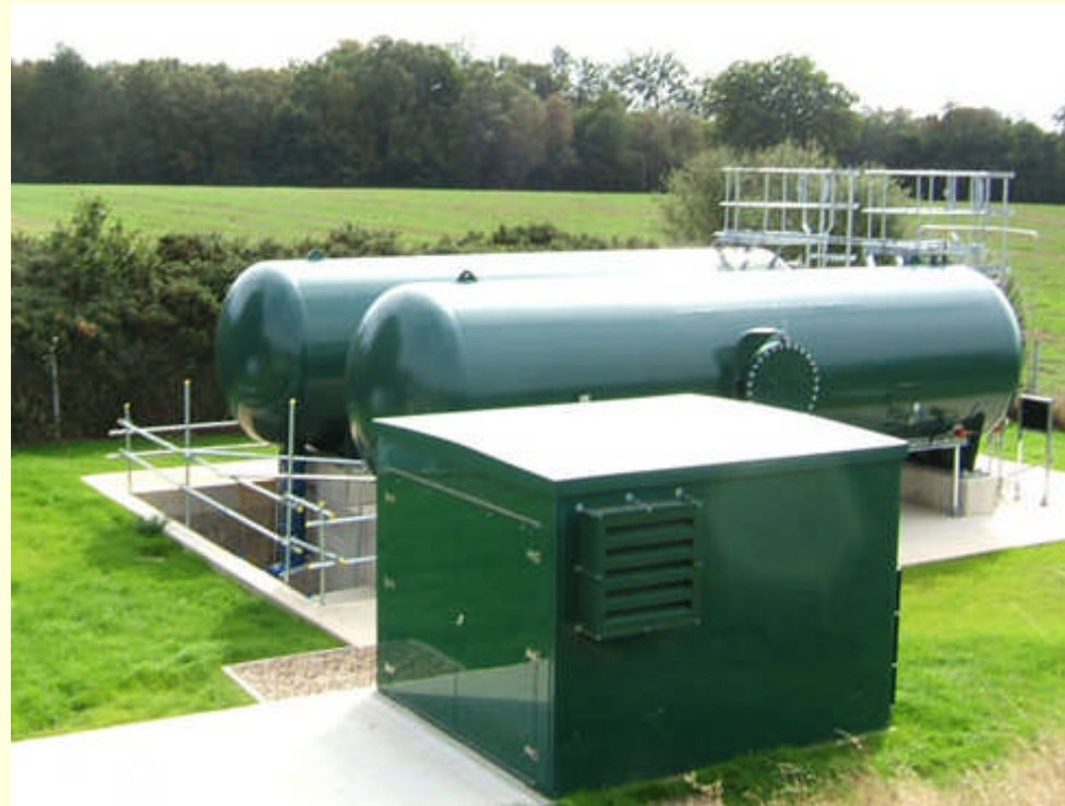
Horizontal Air chamber for water hammer prevention
