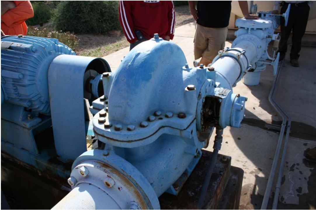
Split-Case centrifugal pump.
