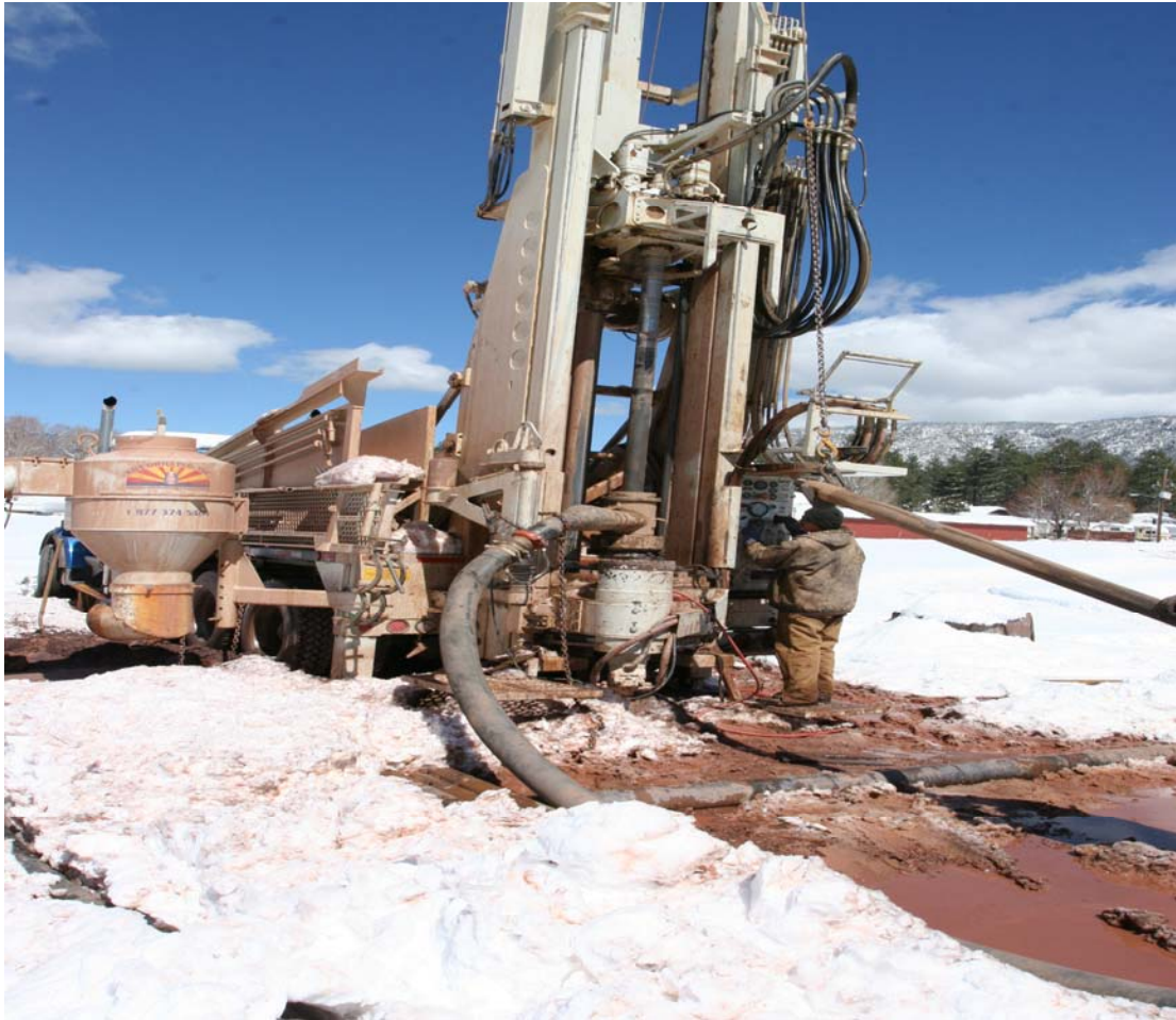
A drill rig in the snow.
