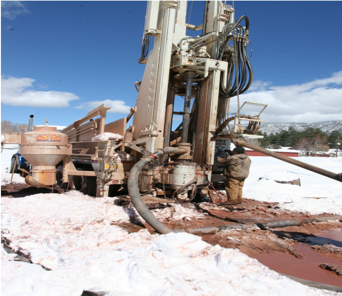
A drill rig in the snow.
