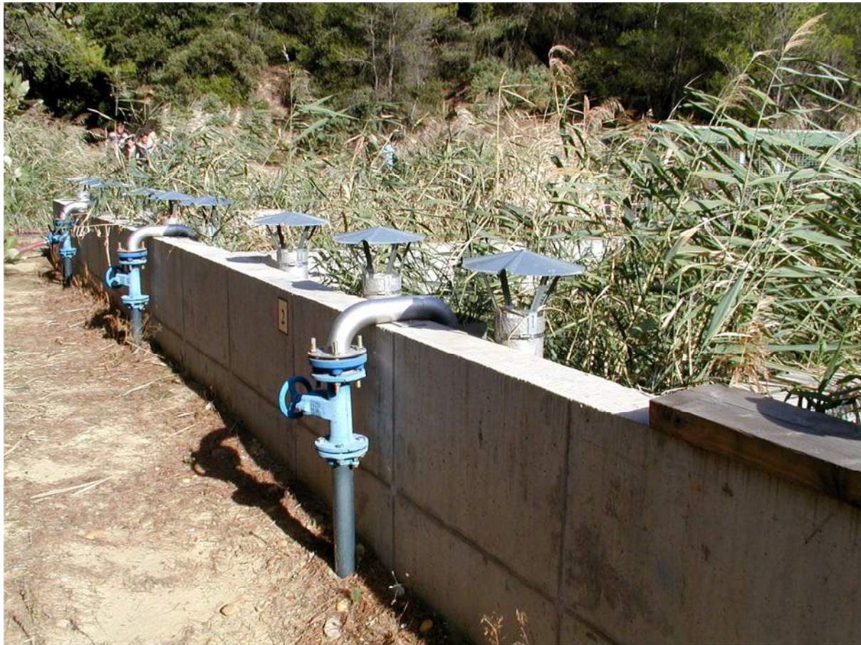
Photo 31: Arrangement Sludge Basins with Wetland Plants (France)
