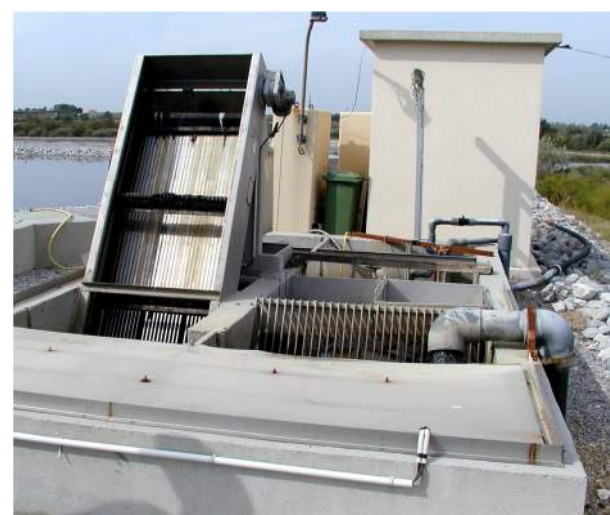
Photo 3a,b: Mechanically Raked Screens
