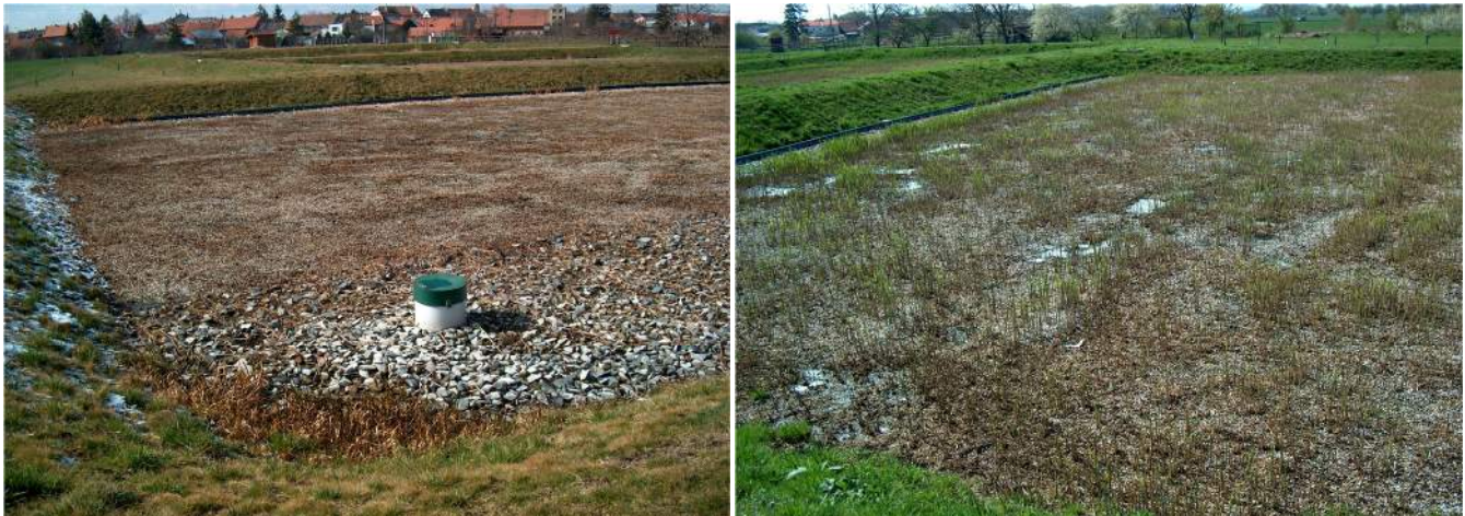
CTW at Čehovice (CZE) – reed during spring period approximately one month after burning old growth (left) – constructed wetland filters after burning of old growth of reed in March – old vegetation is burned outside the constructed wetland filters (right)
