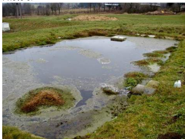
Photo 6: Small Settling Tank Overgrown with Filamentous Algae
