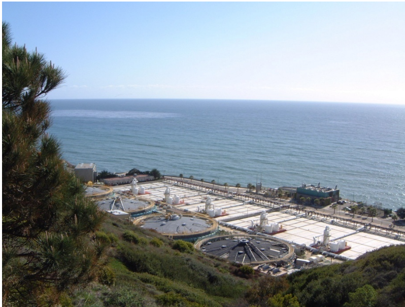
Aspect of Sewage plant
